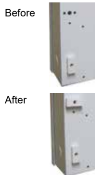
Figure 2a: Installing plastic spacer
