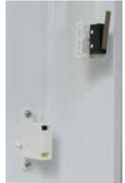
Figure 2b: Installing the tamper switches
