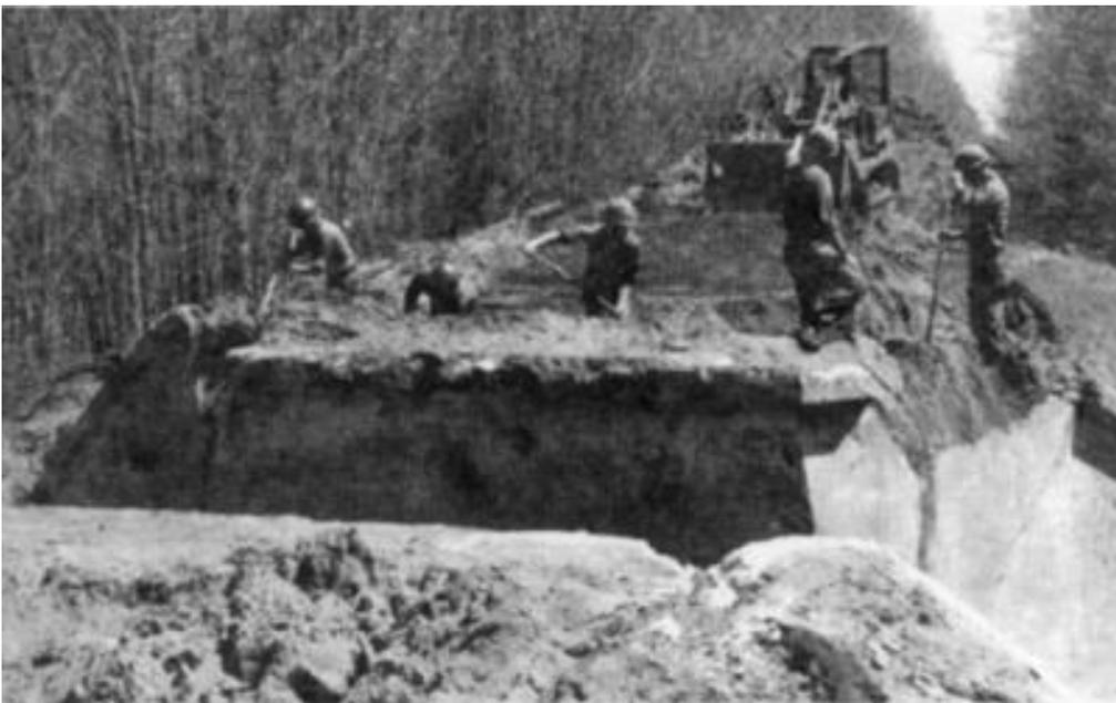
The Battalion is still a "combat" battalion. After carefully installing the demolition charges, an engineer squad "cooks them off" and completely destroys a set of bridge abutments. Credit: SP4 Ron Hess
