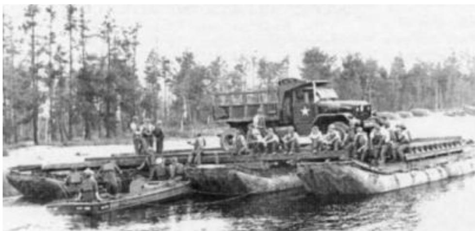
Although the M4T6 raft is considered technologically obsolete, large stocks of the bridge assure its wartime use, and they require the 107<sup>th</sup> to continue to be proficient in its construction. Credit: SP4 Ron Hess
