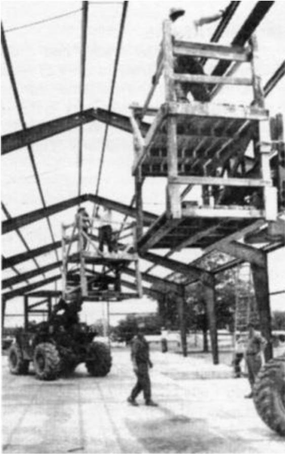
The Battalion construction section has a limited construction capability. Above, they are assembling a steel warehouse at Camp Grayling.
