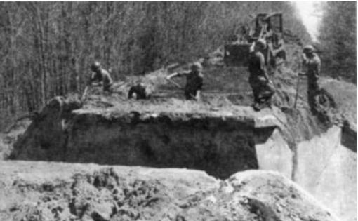
The Battalion is still a "combat" battalion. After carefully installing the demolition charges, an engineer squad "cooks them off" and completely destroys a set of bridge abutments. Credit: SP4 Ron Hess
