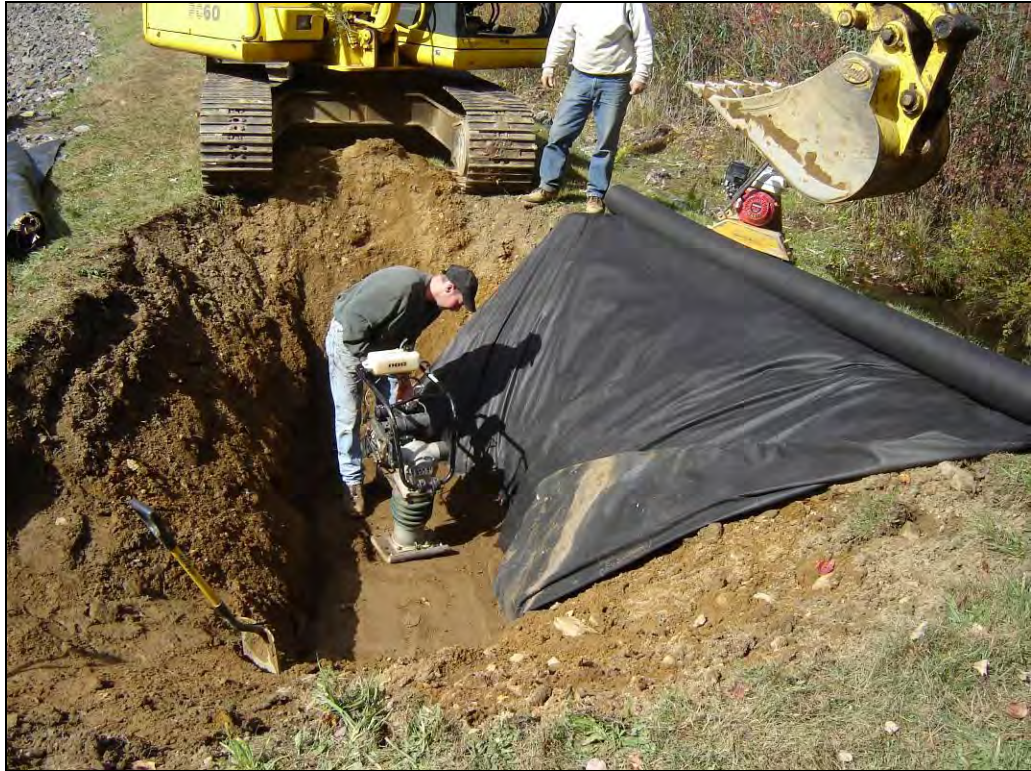
Photo 9: Embankment fill placed and compacted in 8-inch lifts (1 of 4)
