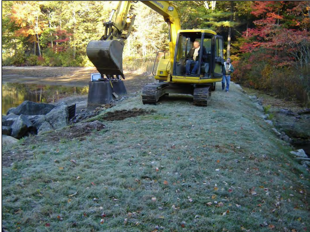
Photo 3: Start of excavation
