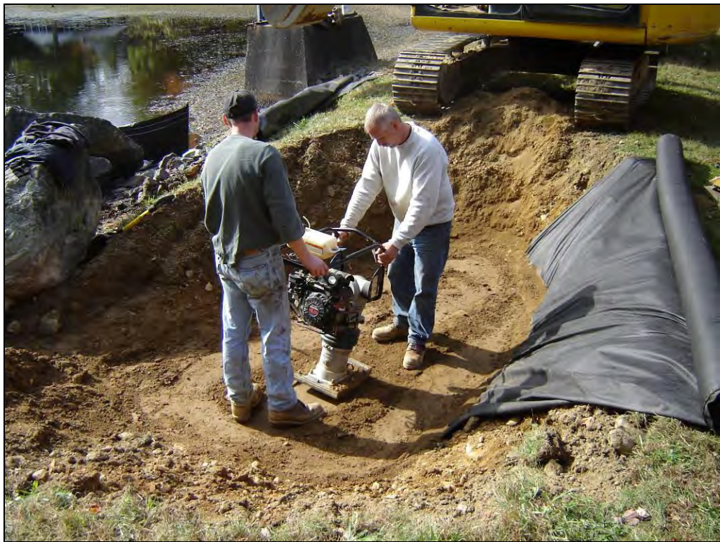
Photo 10: Embankment fill placed and compacted in 8-inch lifts (2 of 4)
