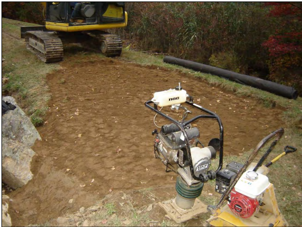
Photo 12: Embankment fill placed and compacted in 8-inch lifts (4 of 4)
