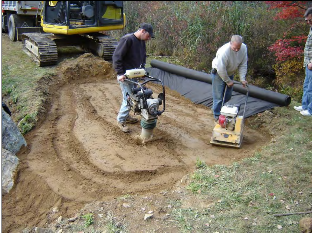
Photo 11: Embankment fill placed and compacted in 8-inch lifts (3 of 4)
