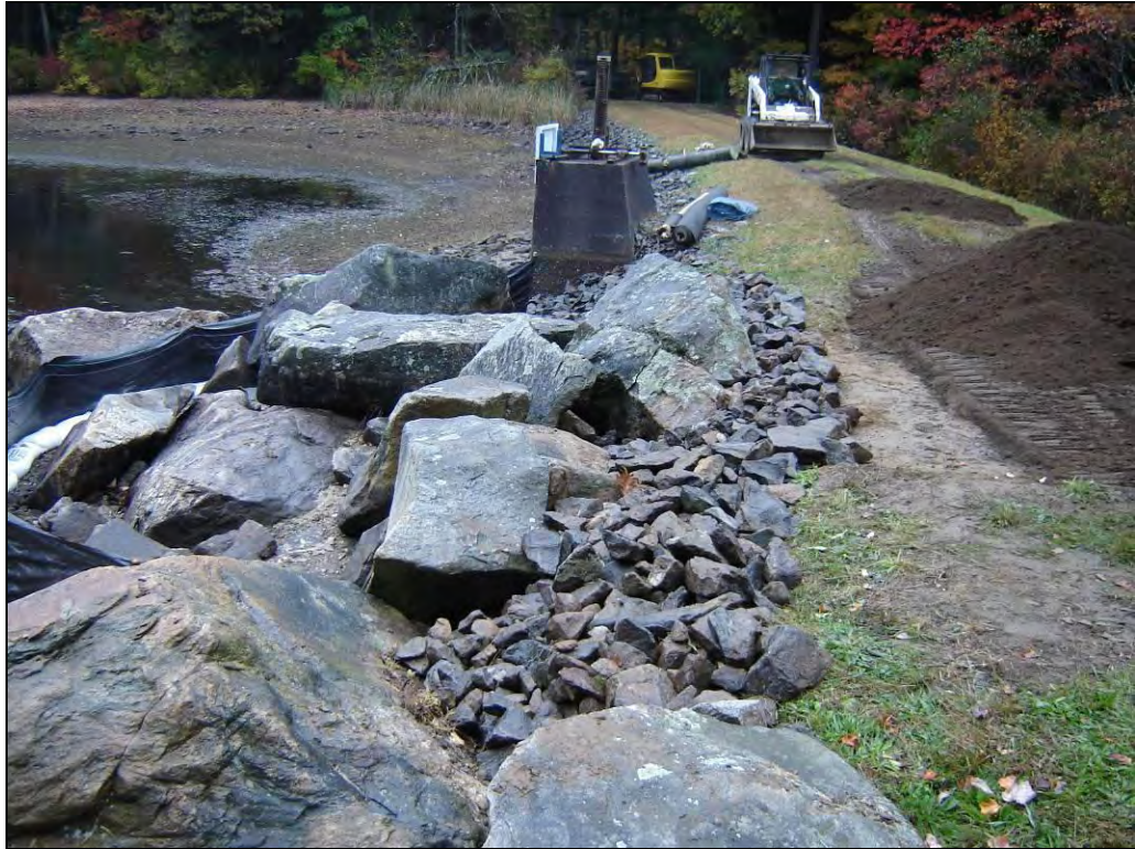
Photo 13: Riprap re-installed along the dam's upstream face for erosion protection
