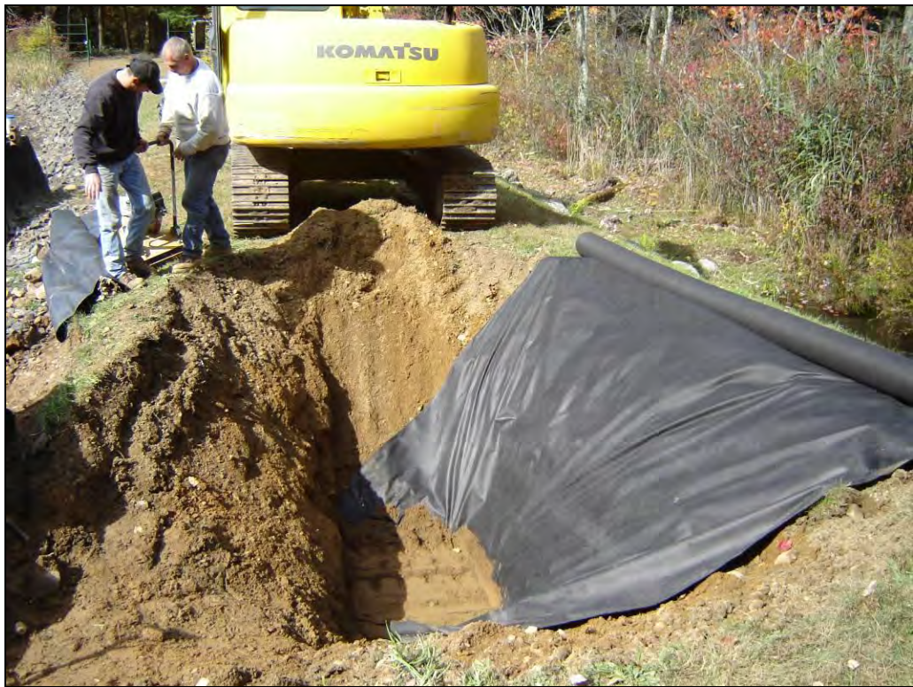
Photo 8: Permeable filter fabric installed, lining the downstream face of the excavation.
