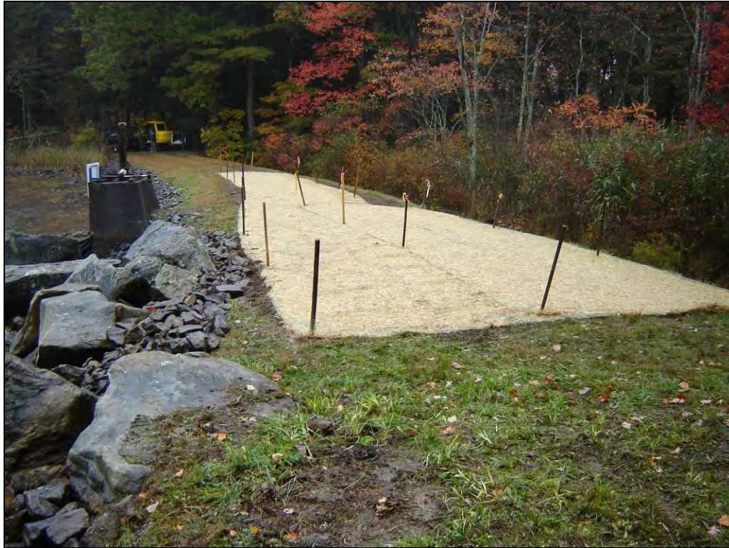
Photo 15: Hay matting placed and staked for erosion protection.
