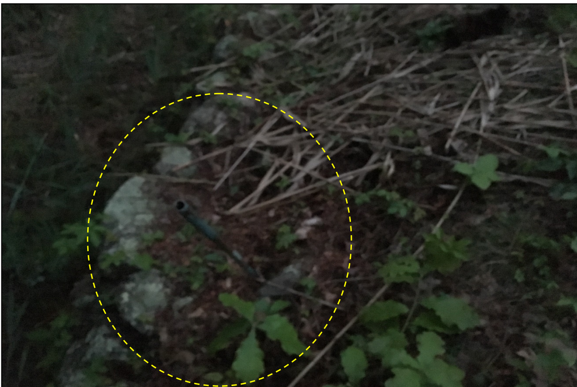
Photo 24: Areas of specific deficiencies – depressions at the downstream side of the crest.
