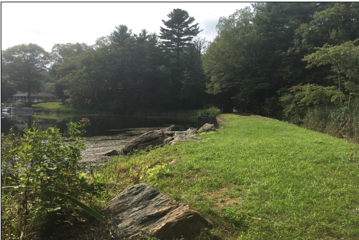
Photo 2: Overview of upstream face from right abutment.
