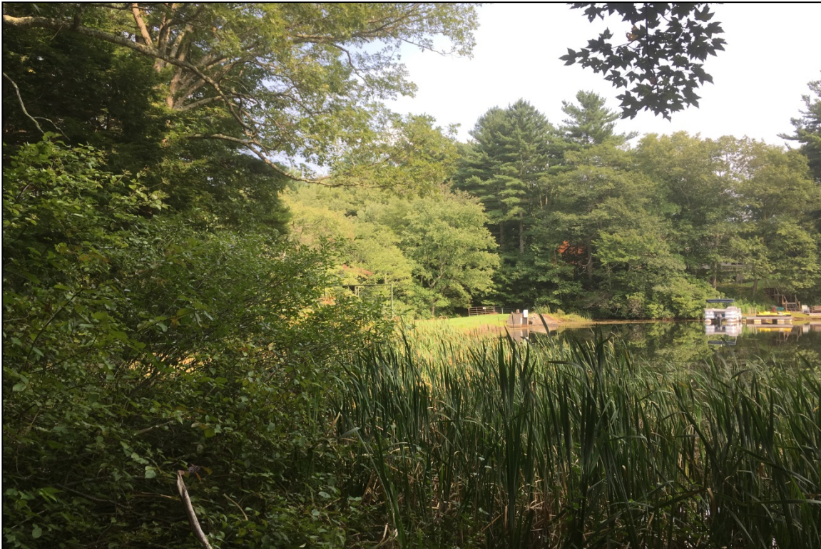
Photo 1: Overview of the dam from upstream
