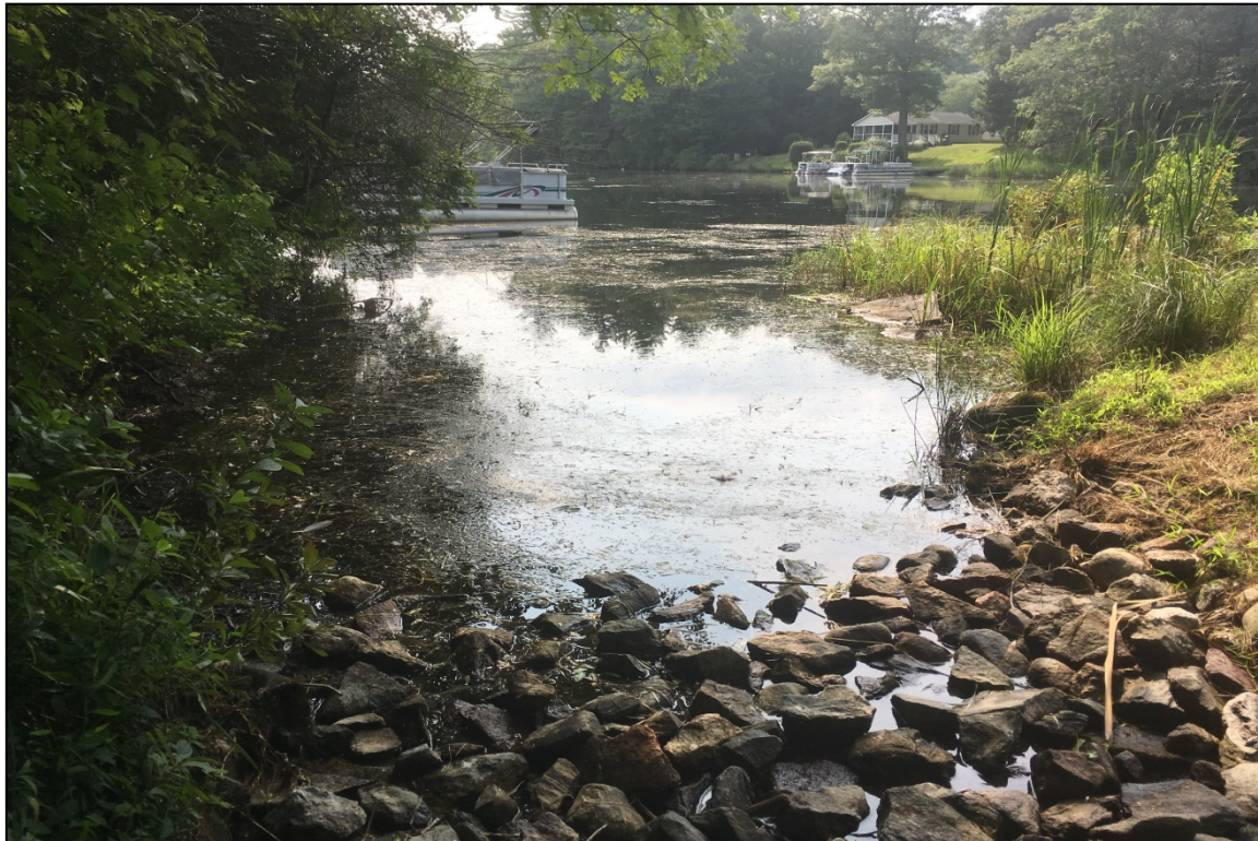
Photo 19: Overview of reservoir area.
