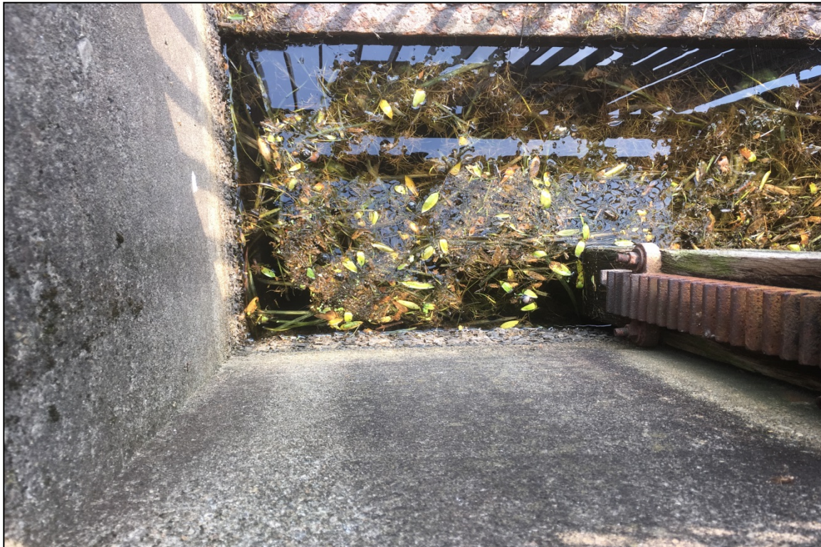
Photo 9: Overview of primary spillway/low level outlet interior.
