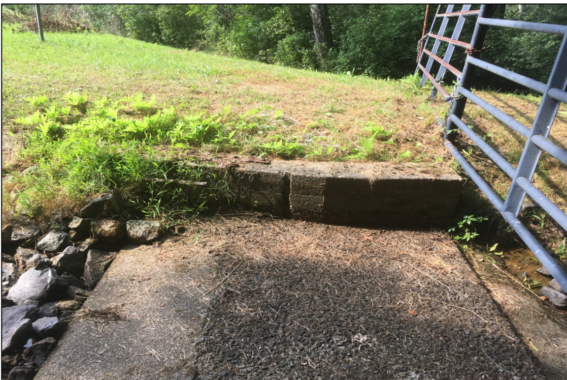
Photo 16: Overview of left training wall.
