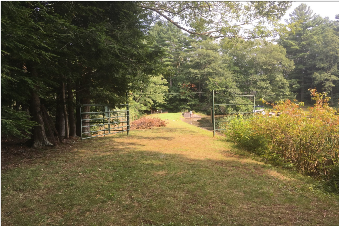
Photo 5: Overview dam crest from left abutment.
