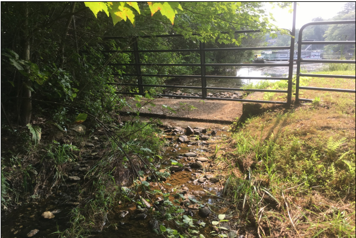
Photo 14: Overview of auxiliary spillway from downstream channel area.
