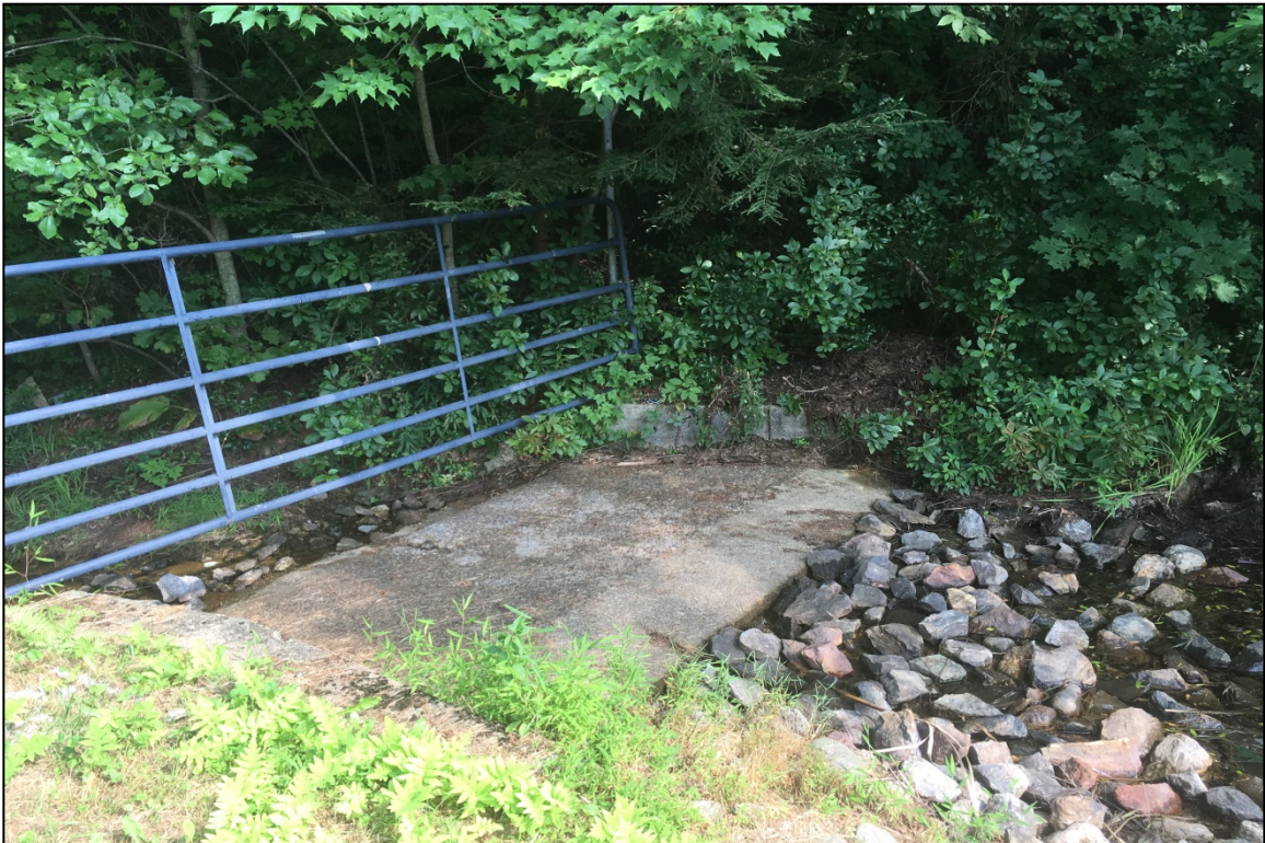
Photo 13: Overview auxiliary spillway from the left side of the spillway.
