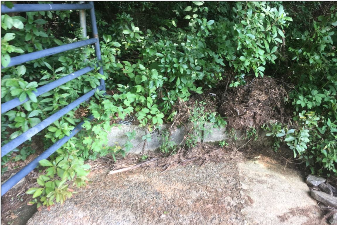
Photo 15: Overview of right training wall.
