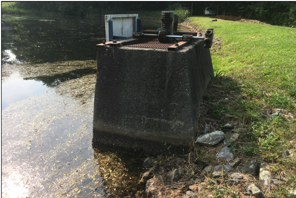
Photo 8: Overview primary spillway from the right side (Owner uses low level outlet as the primary spillway).
