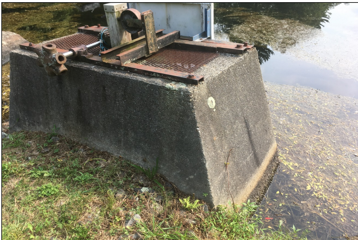
Photo 10: Overview of primary spillway/low level outlet exterior.
