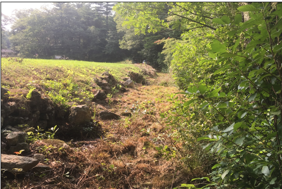
Photo 6: Overview of downstream face from right abutment
