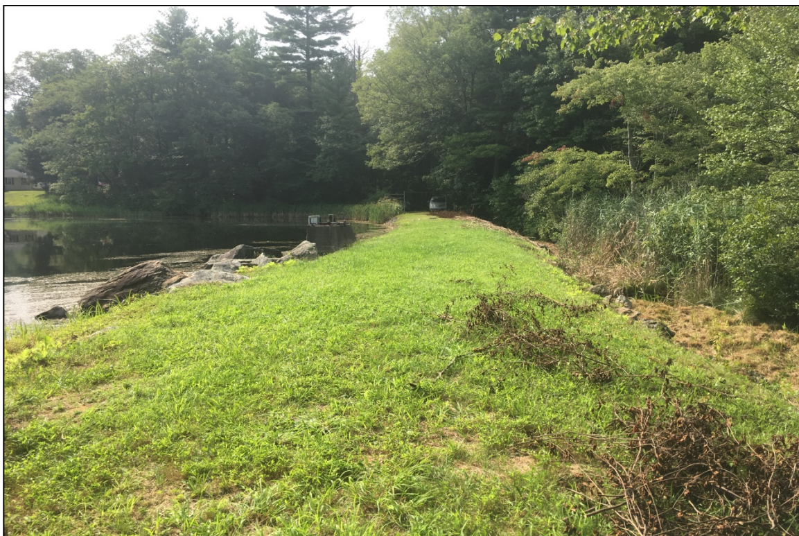
Photo 4: Overview of dam crest from right abutment.
