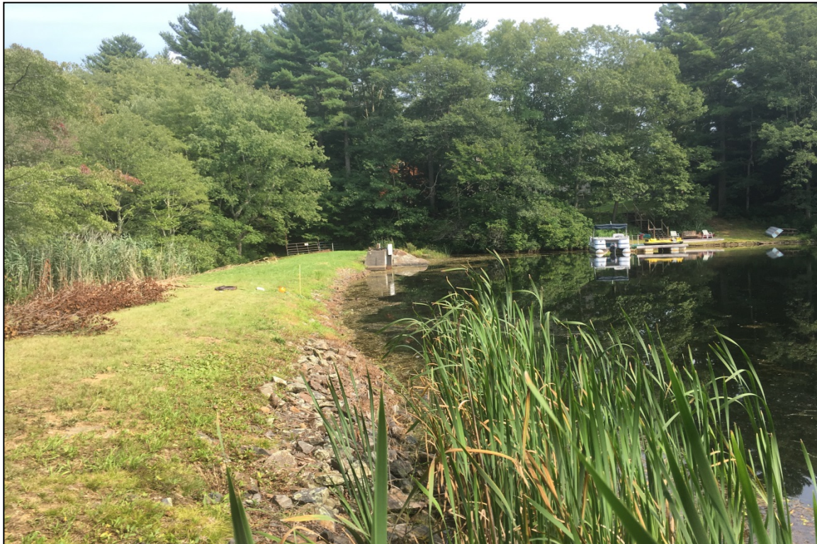
Photo 3: Overview upstream face from left abutment.
