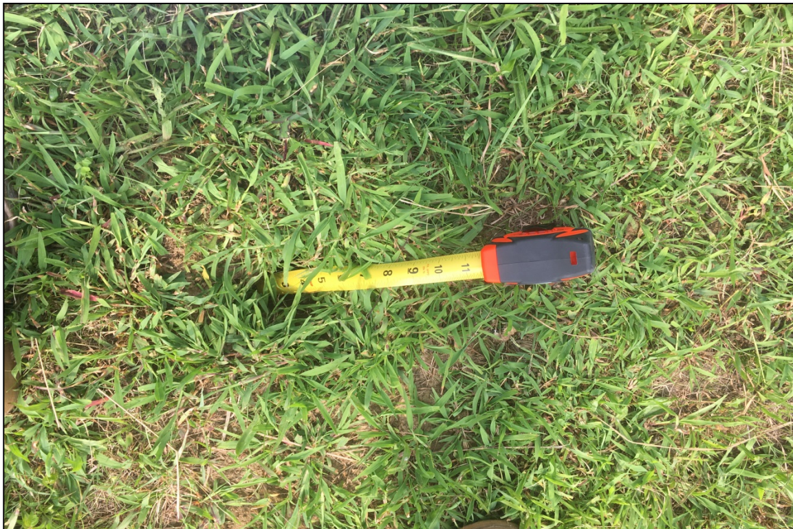
Photo 20: Areas of specific deficiencies – Rodent hole on the crest (typ.).
