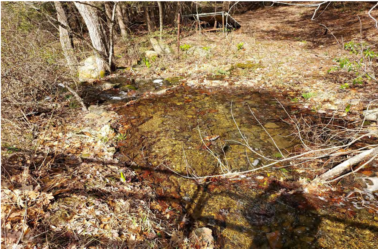
Photo 15a – The immediate spillway channel area downstream of the spillway.
