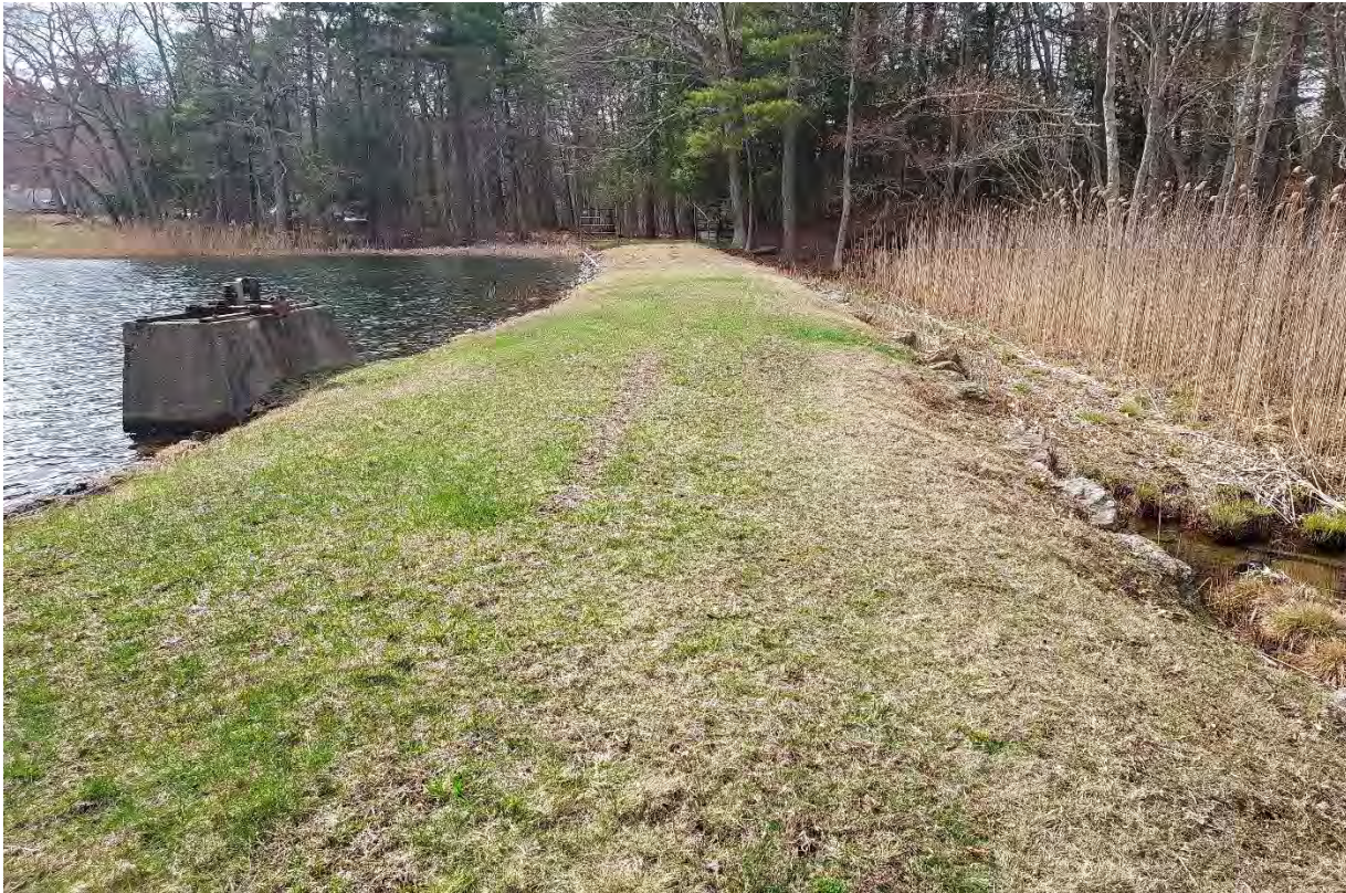
Photo 5 – The dam crest, taken from the right side abutment.
