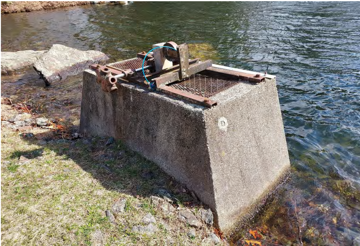
Photo 16a - The exterior of the gate control structure, seen from its left downstream side with Crystal Pond to the right.
