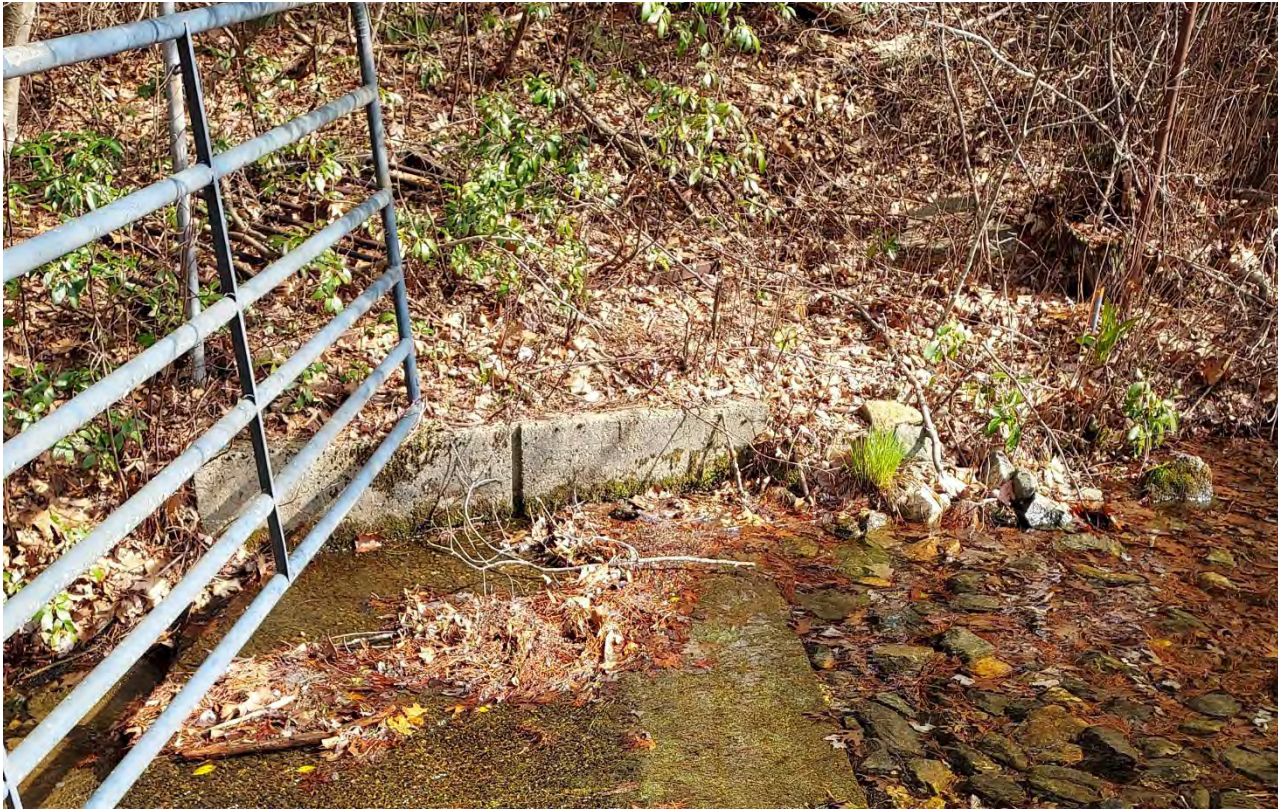
Photo 11 – The short section of the right side spillway training wall.
