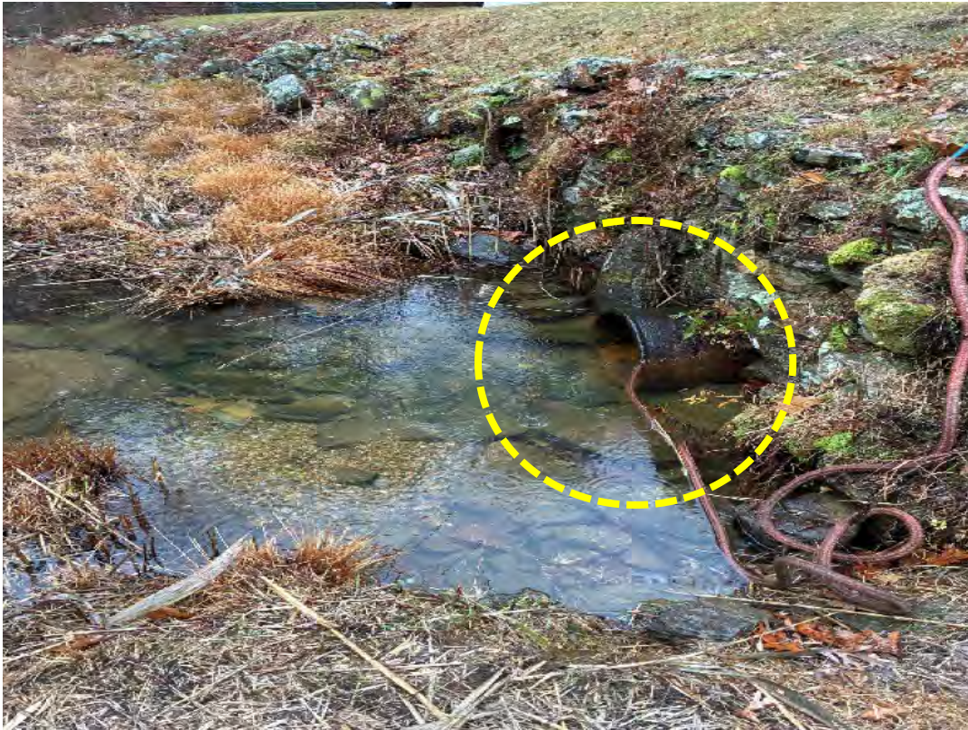
Photo 19a – The discharge point of the 24-inch cast iron low level outlet pipe on the downstream embankment slope, taken during the outlet structure's repair.
