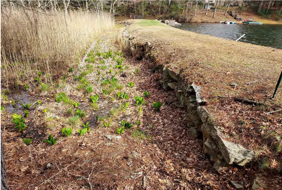
Photo 8 – The downstream face of the dam, seen from the left side abutment.
