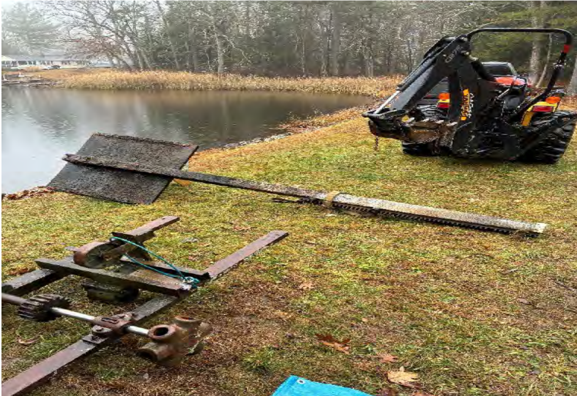
Photo 18 – A view of the gate operator, at bottom left, taken during the structure refurbishment noted in the previous photos.
