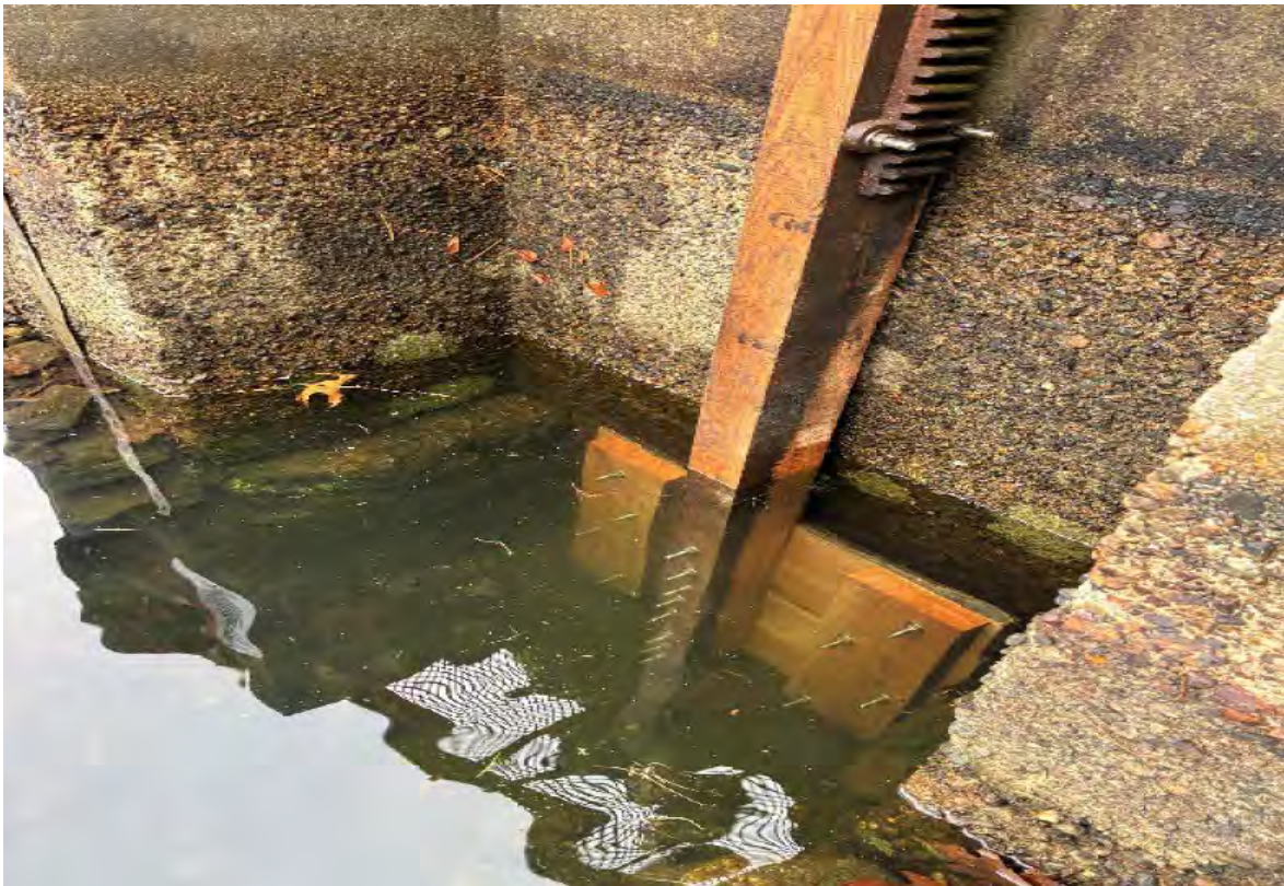
Photo 17 – The interior of the intake / outlet gate control structure, seen from its upstream side while under reconstruction during November of 2025.
