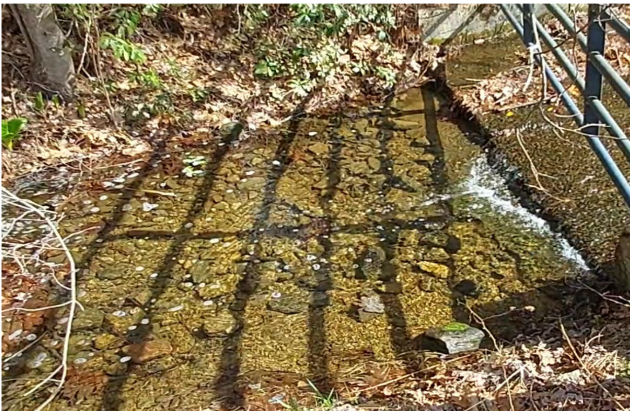
Photo 14 – The sloped stilling basin area, just downstream of the spillway apron.
