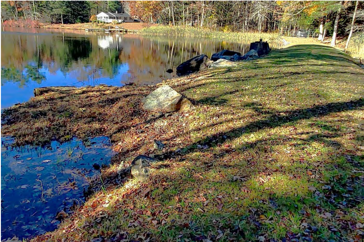
Photo 1 - The upstream side of the dam as seen from its right side.
