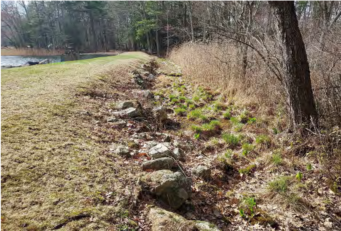
Photo 7 – The downstream face of the dam, taken from the right side of the dam.
