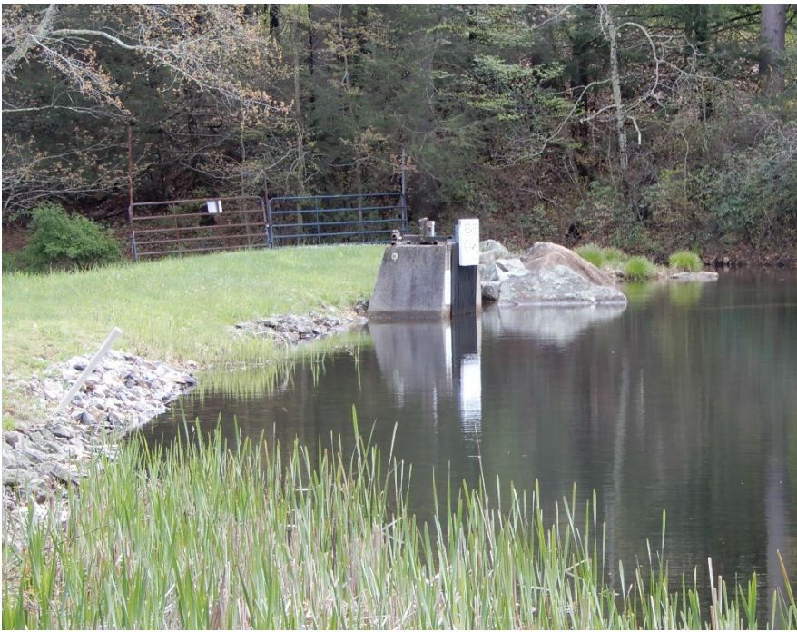
Photo 2 – Riprap along the upstream shoreline of the dam on the left side and a mix of large rocks and small boulders on the right side.
