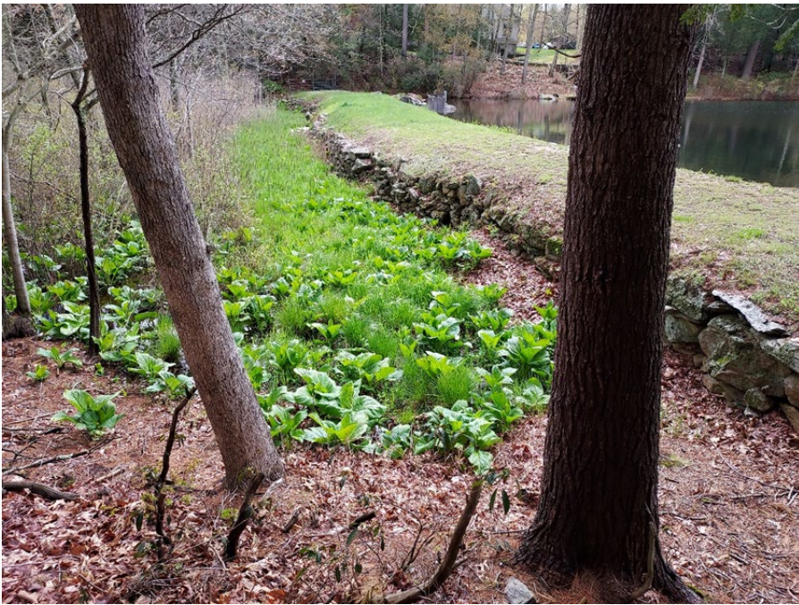
Photo 4 – The downstream slope, as seen in this view from the left side looking toward the right side. Note that, as with the previous view, there is an extensive marshy area directly at the base of the dam and extending northward therefrom.
