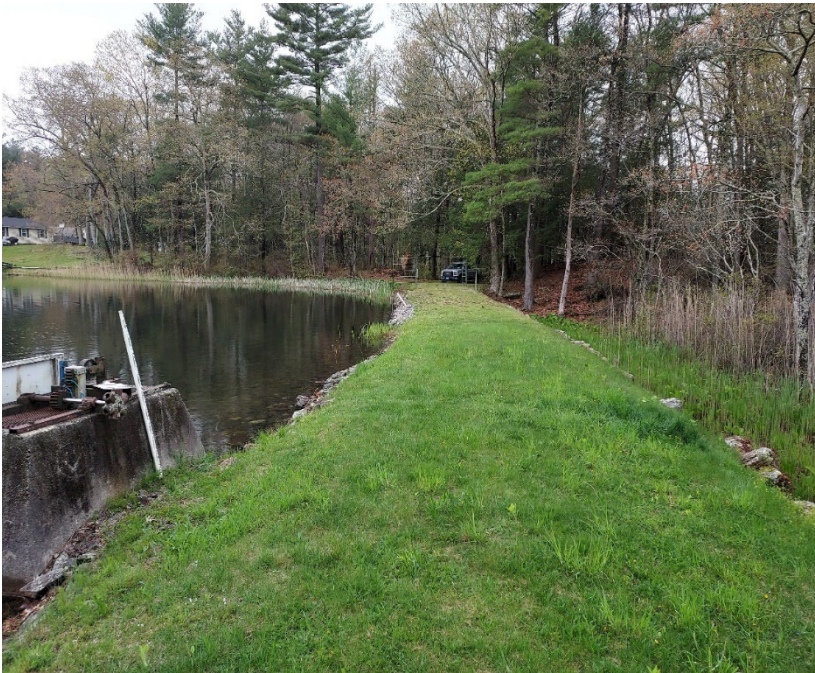
Photo 1 – The crest as seen from the right side of the dam looking toward the left side.
