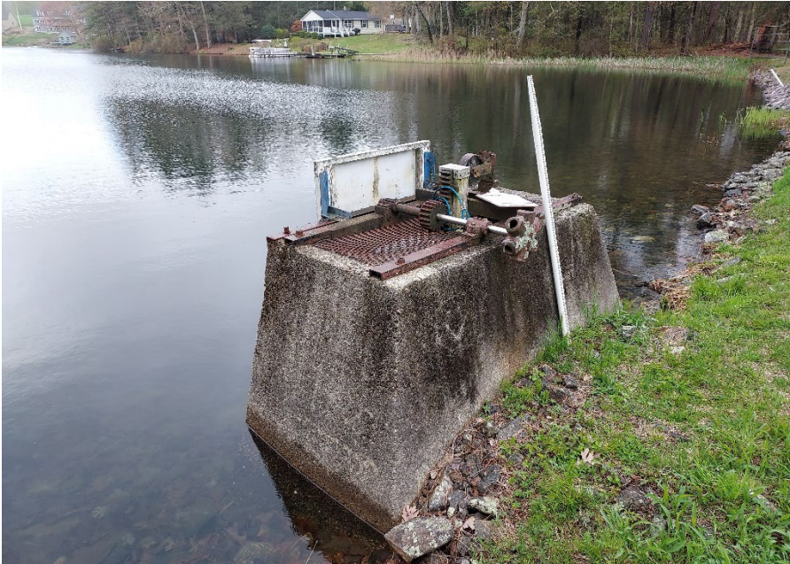
Photo 6 – The gate structure as seen from its right side.
