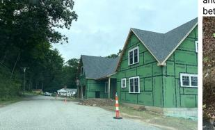
Home construction not using adequate soil and erosion control practices. Contractors should prevent tracking soil onto the road and install silt fences to prevent erosion of open soil.
