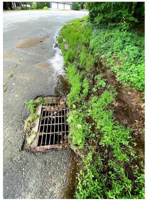
Would be best to discourage property owners from storing large amounts of open sediment near the side of the road. Machinery can easily track soil into the road, bringing large amounts of phosphorus attached to soil particles that will eventually get washed into the catch basin system during rainfall events.
