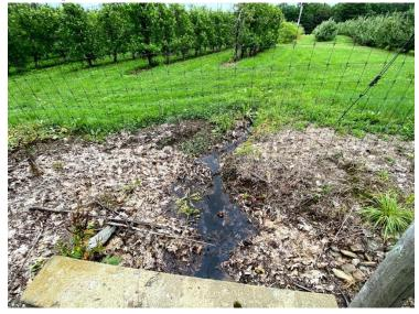
**Soil erosion just uphill of Inlet (Culvert) 9 on Lake Drive**, just around the corner from Crystal Pond Road private property runoff from construction land disturbance – could use catch basin filters to prevent sediment from flowing into the basins during high-flow storms. (41.918475, -72.105042)
