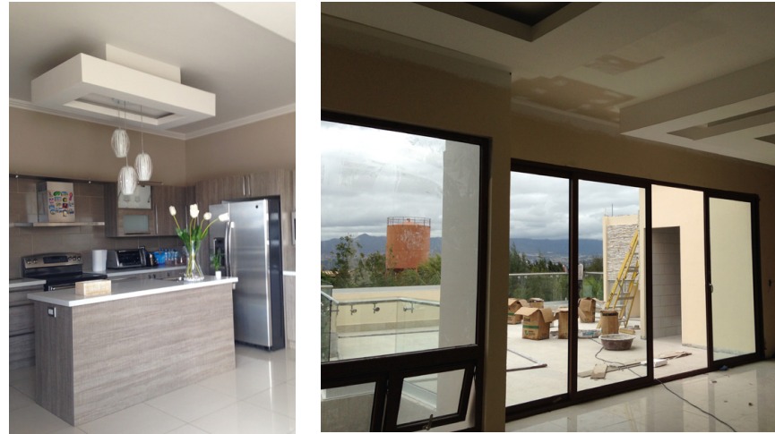
Kitchen Cabinetry Design Livingroom/kitchen in process of construction
