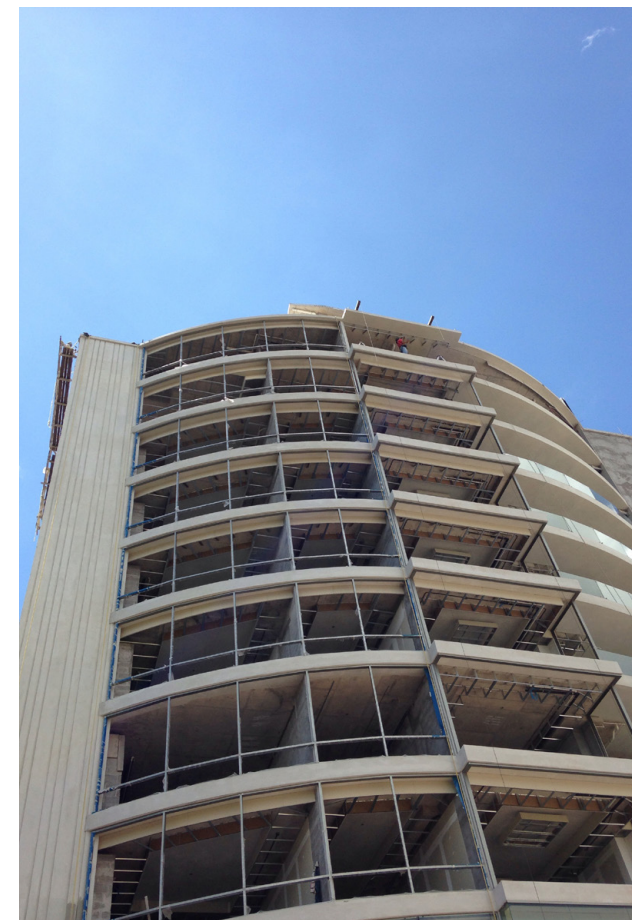
Process of construction of main facade..
