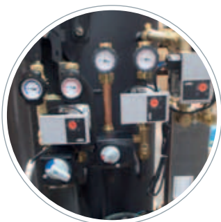
Heating circuit distributor
