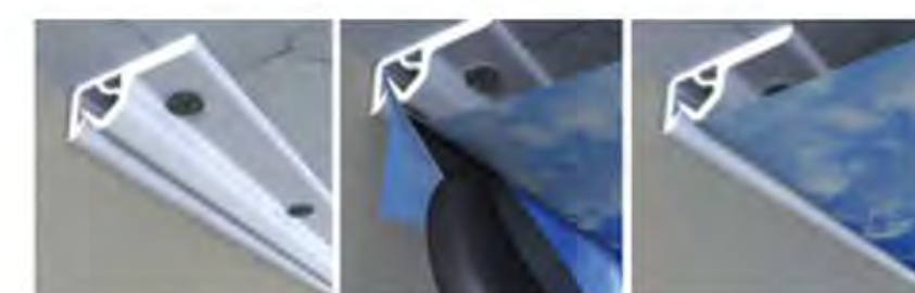
1. Attach Profiles 2. Tuck Fabric 3. Stretch and Trim
