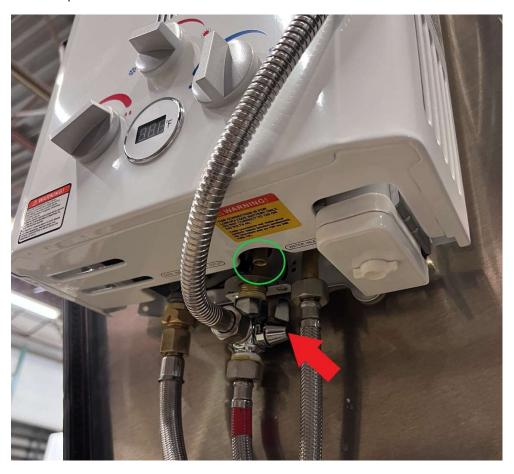
Step 7: Ensure all water has drained from the tank, if needed, wait for tank to completely drain before moving on to the next step.
