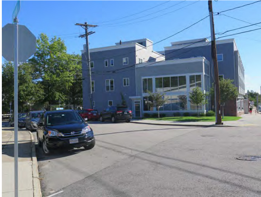
View of Mixed-Use Building on other side of Anawan Avenue
