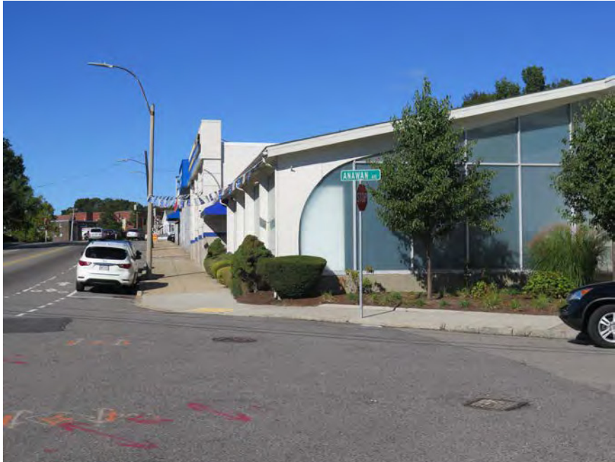
View of Existing Buildings from Anawan Avenue.
