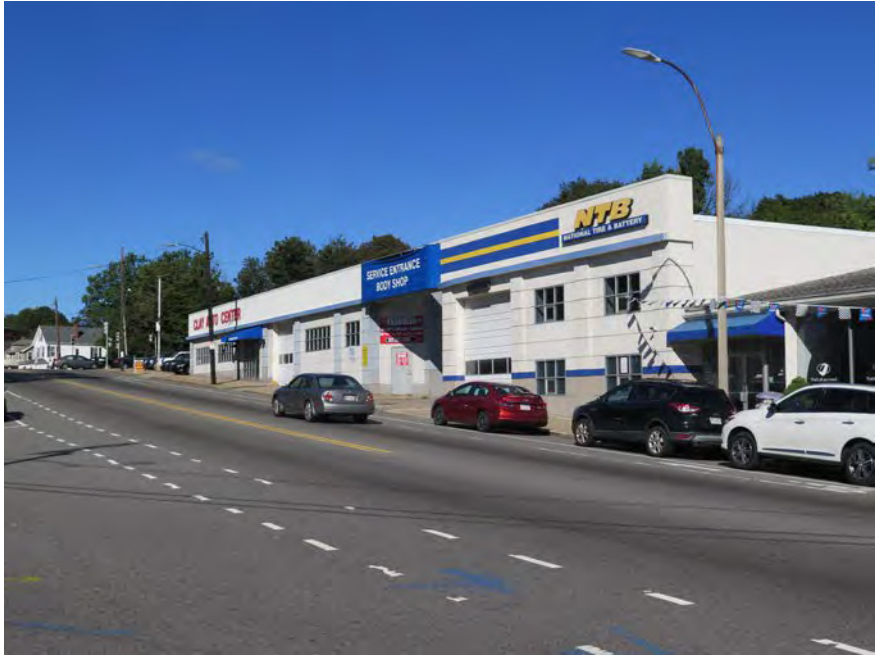
View of Existing Buildings from Belgrade Avenue.
