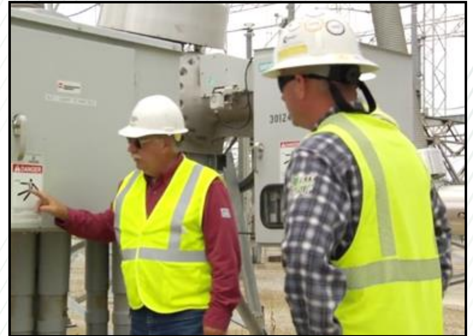
Referencing Voltage On The Cabinet
