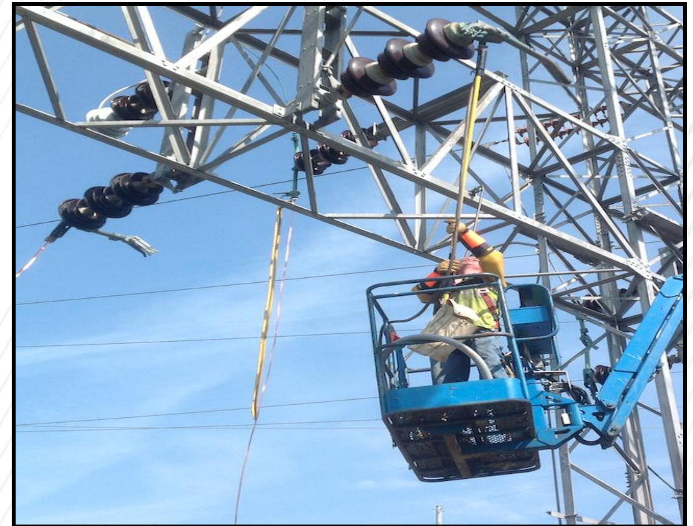
Employee Maintaining MAD With Insulated Hot Stick
