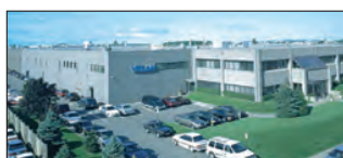
Montreal, Canada Velan Inc., Plant 2 and 7
