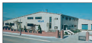
Ansan City, South Korea Velan Ltd., Plant 1
