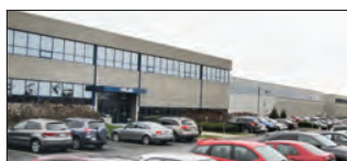
Montreal, Canada Velan Inc., Plant 5
