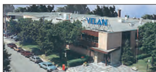
Montreal, Canada Velan Inc., Plant 1
