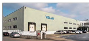
Ansan City, South Korea Velan Ltd., Plant 2
