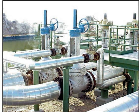
*A geothermal power plant valve installation for sour gas service.*
