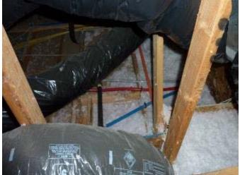
Portions of the polyethylene supply piping were exposed to sunlight in the attic. Over time the cross-linked polyethylene piping could become damaged by the sunlight coming through the attic vents. We recommend the piping be covered by insulation as preventive maintenance.
