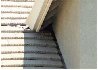
A roof tile at the left side of the dormer has slid out of place. We recommend the tils be repositioned and resecured by a qualified roofing contractor.
