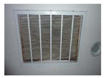
The filter had accumulated debris that decreased its effectiveness and blocked airflow. This condition can dramatically decrease the efficiency of the system, decrease the service life of the furnace and increase maintenance costs. A properly sized new replacement air filter should be installed and secured in the correct orientation in this unit.
