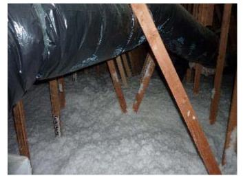
The insulation had settled or had been compressed and no longer provided the same R-value as when it was installed. At the least, additional insulation should be installed to restore the original thermal efficiency of the attic. Even better would be to add insulation to bring the level up to current industry standards.
