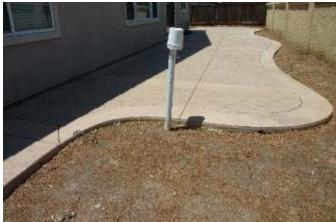
A drain pipe extends well above grade and will not be effective for drainage. We recommend the pipe be lowered to grade and a drain grate be installed.
