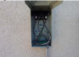
The visible and accessible wiring for the electrical supply was in acceptable condition.
