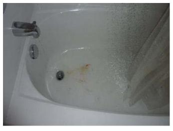
The bathtub was rusted. We recommend repairs be made by a qualified professional.
