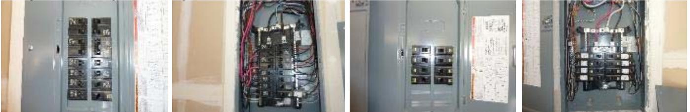
Circuits in each of the subpanels were labeled. The accuracy of the labeling was not verified. When the opportunity arises, we recommend verifying the accuracy of the labeling by actually operating the breakers.
