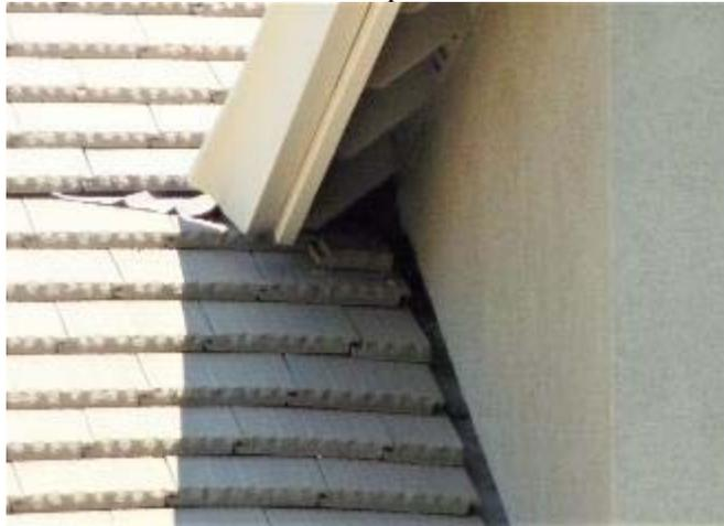
**A roof tile at the left side of the dormer has slid out of place. We recommend the tiles be repositioned and resecured by a qualified roofing contractor.**
