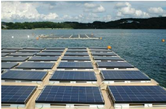
Figure 6: System in Aichi, Japan. 2x 10kWp, one water cooled. [7]
