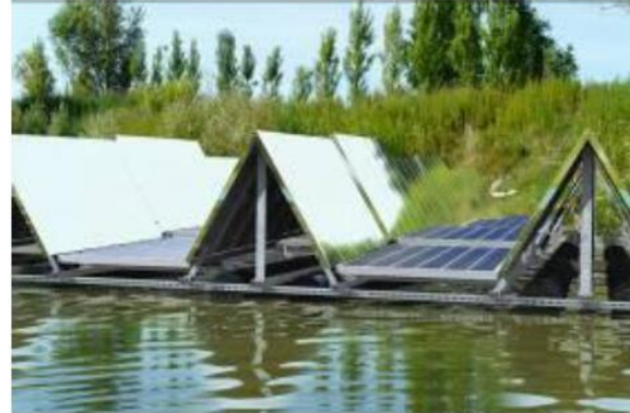
Figure 4: Setup adopted at the Pisa installation with low level concentration. The plant rotates to track the sun's motion [4].
