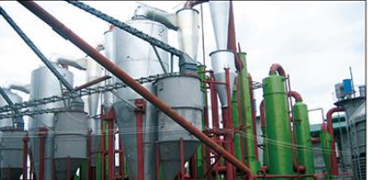
0.5MW CFBG POWER PLANT
