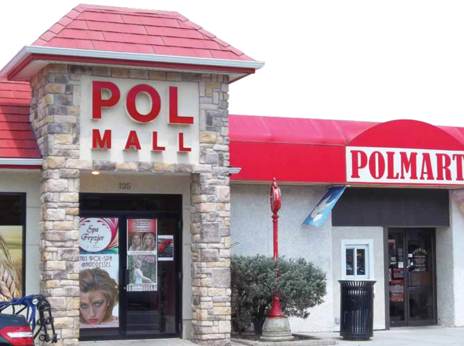
Polmart is the largest Polish themed store on the East Coast. The building houses a bakery, grocery store, deli, hair salon, day spa, retail store, and a fully functioning U.S. Post Office branch. It is the only one in the United States with the word "POCZTA" greeting customers as you enter. (Poczta is Polish for "Post").
