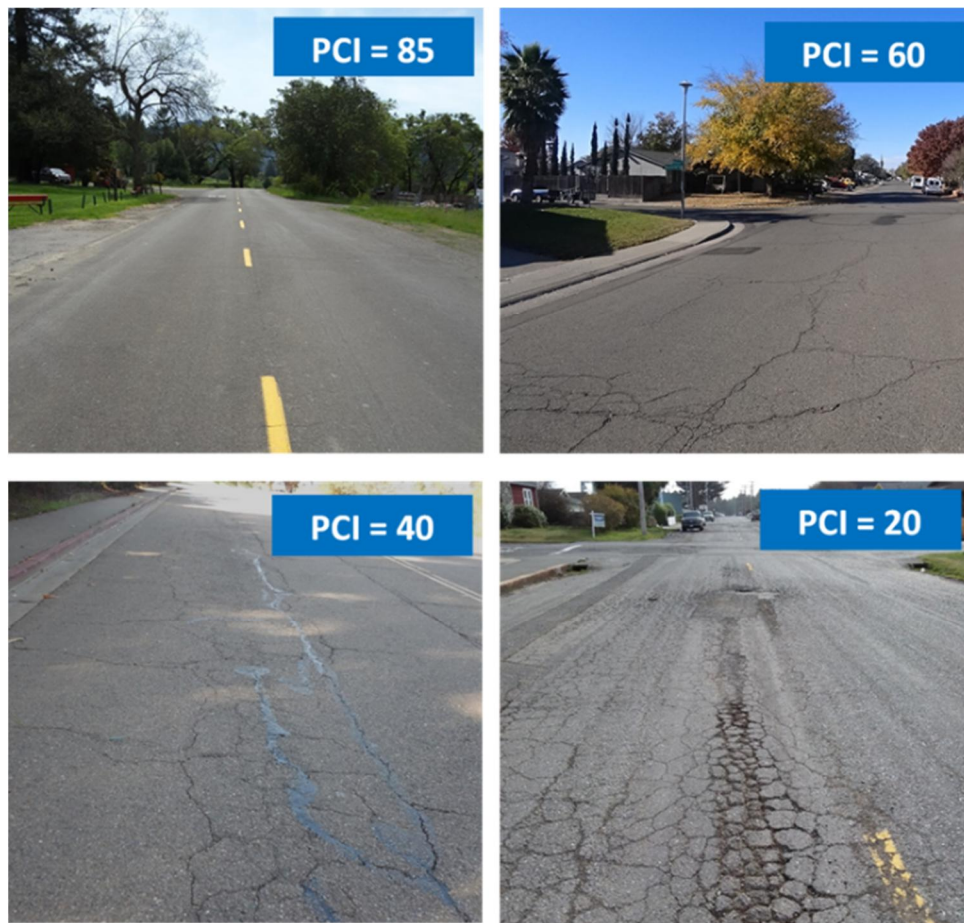
FIGURE 6.1 – Examples of Roadways with Varying PCIs
