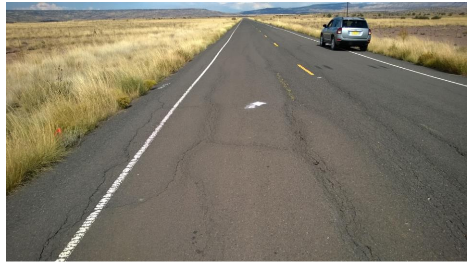
Longitudinal/transverse cracking in location of boring B-19
