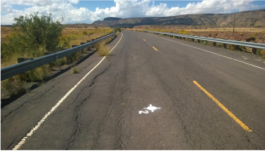
Heaving outside of wheelpath at location of boring B-2
