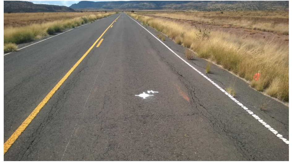
Longitudinal cracking outside of wheelpath at location of boring B-7
