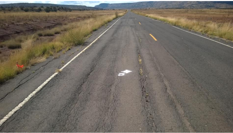
Rutting in wheelpath at location of boring B-10
