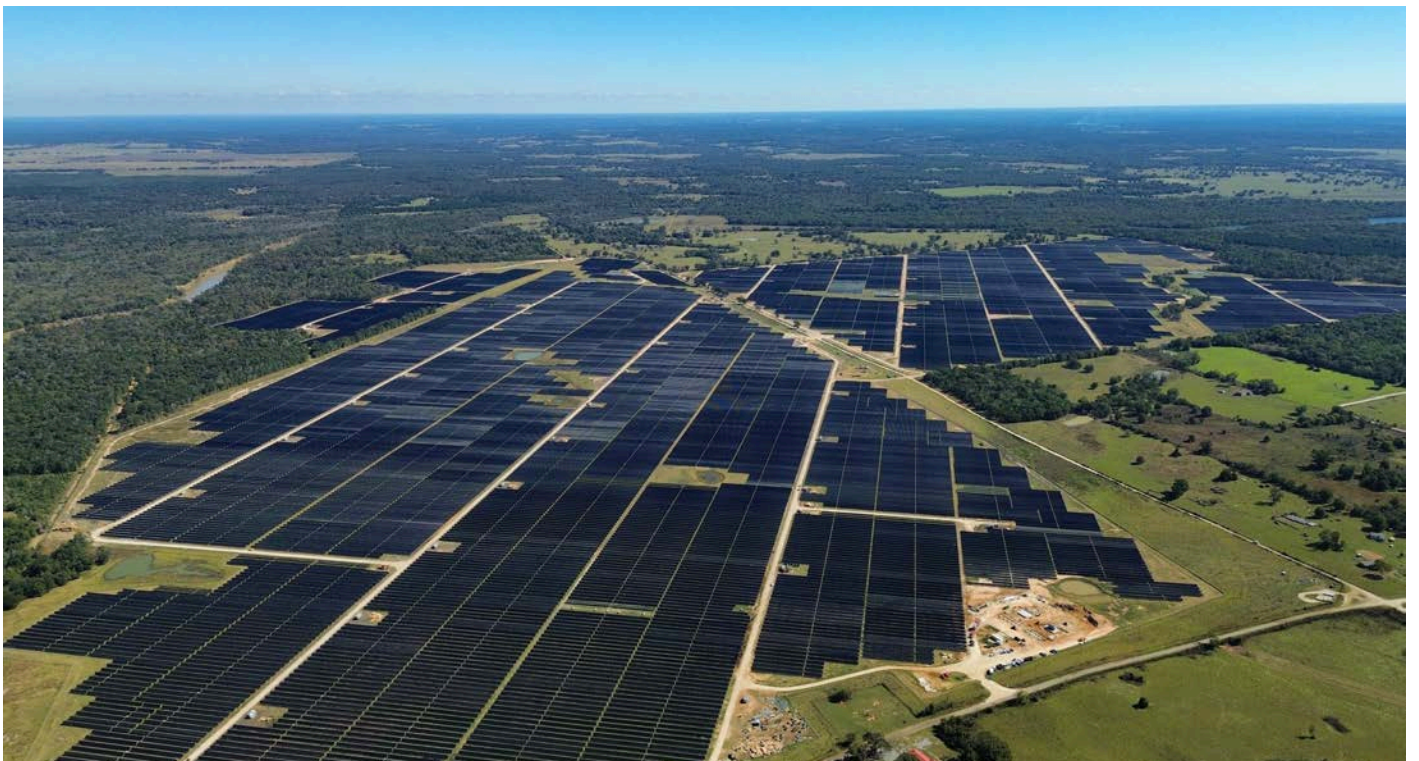
Leon Solar Park (257 MW)
