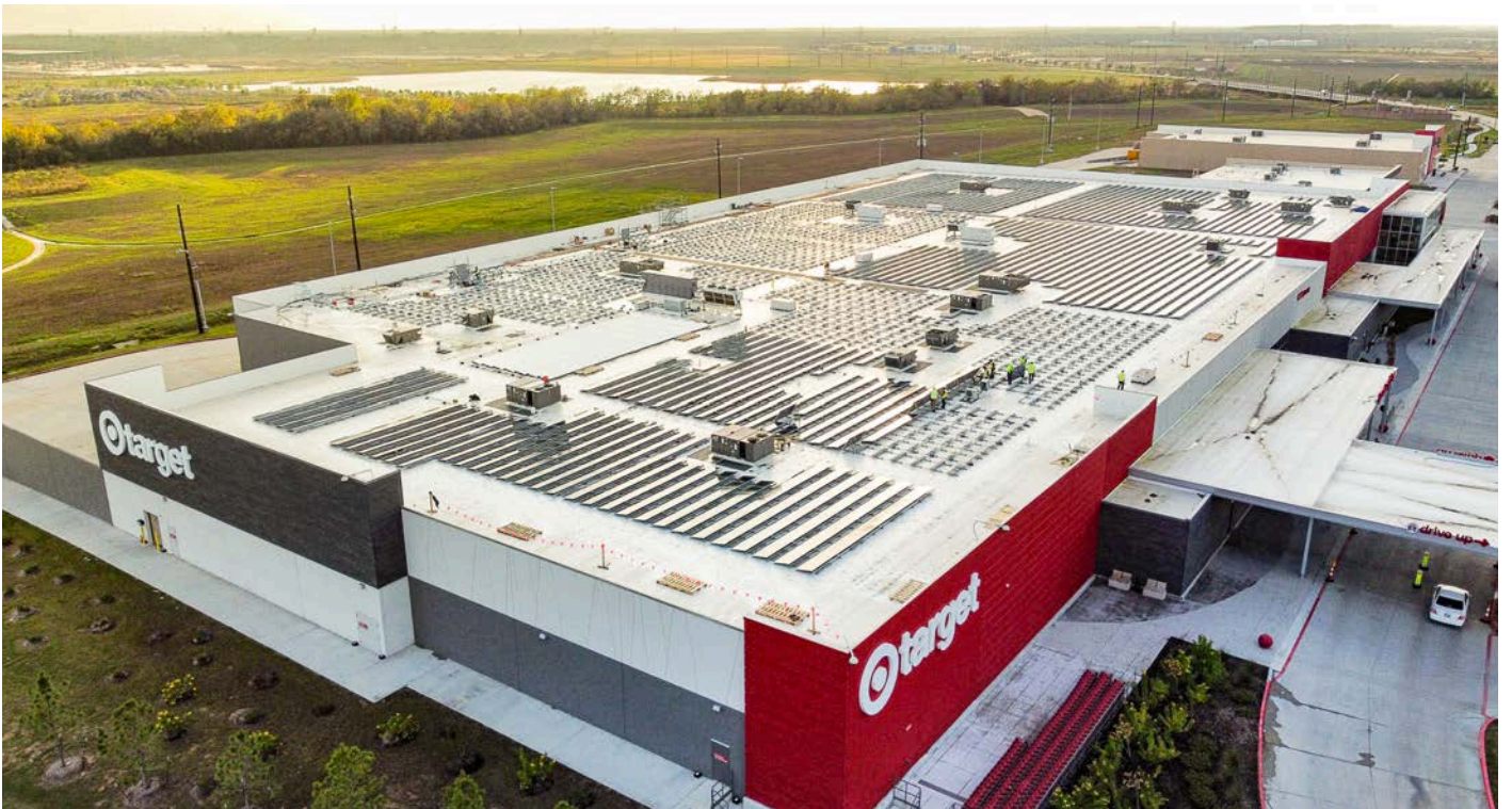
TARGET - Katy, TX (1MW)
