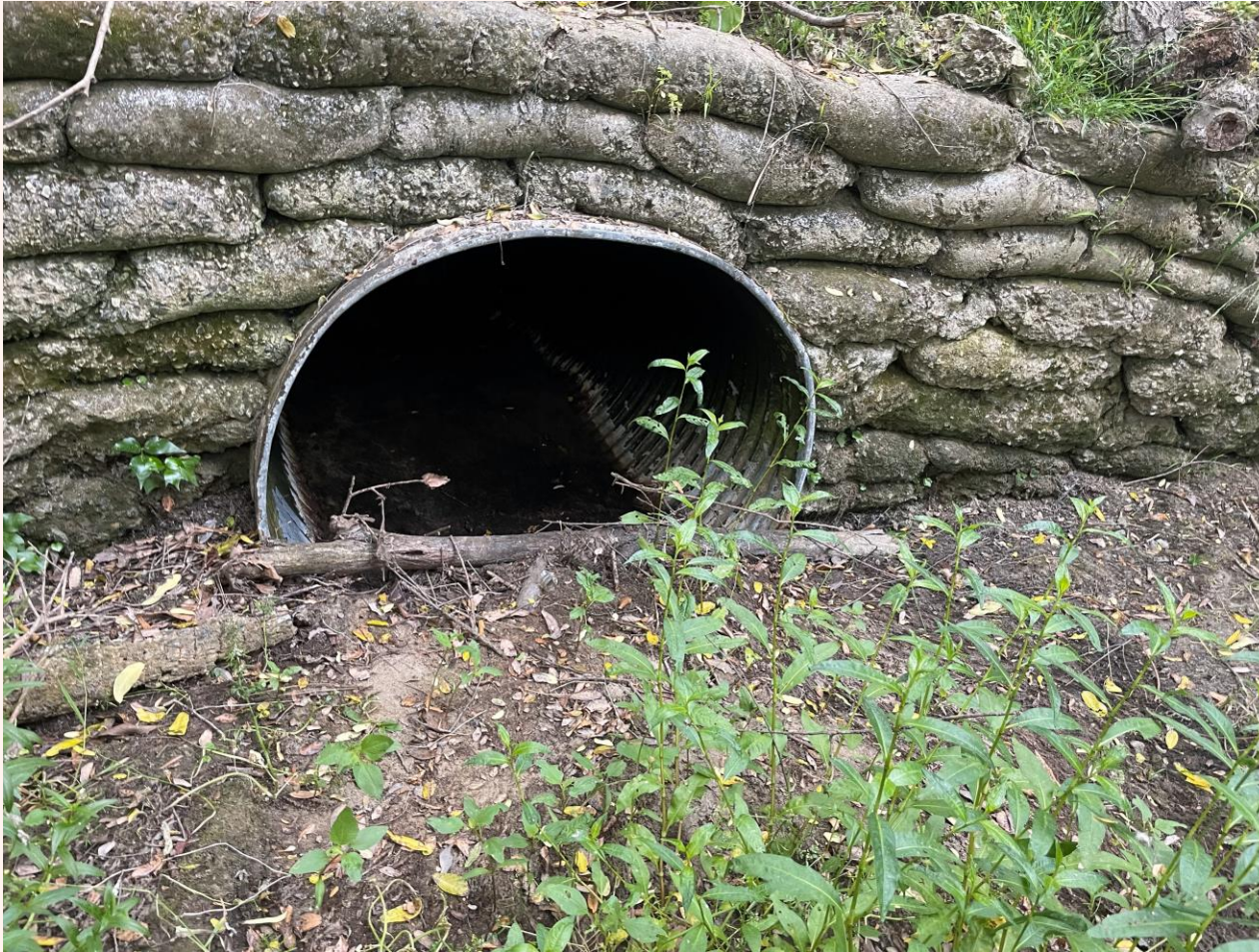
Photo of 48" pipe taken February 2024
