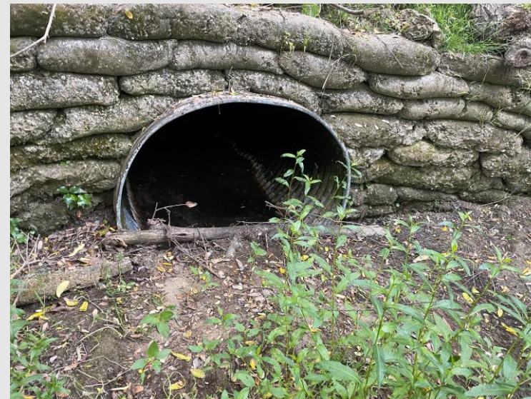
Photo of the 48” corrugated metal pipe and headwall, taken February 2024
