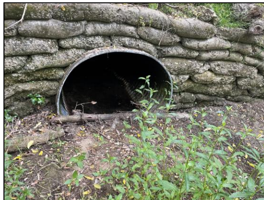
Figure 1 – Photo of the 48” existing pipe and headwall, taken February 2024
