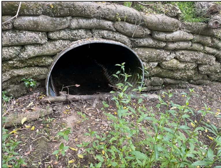
Figure 9 – Photo of the 48” existing pipe and headwall, taken February 2024
