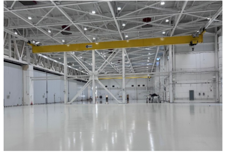
Aircraft Maintenance Hangar, Base Soto Cano Tipo de Cable: THHN/THWN, RHW / EPR, CU
