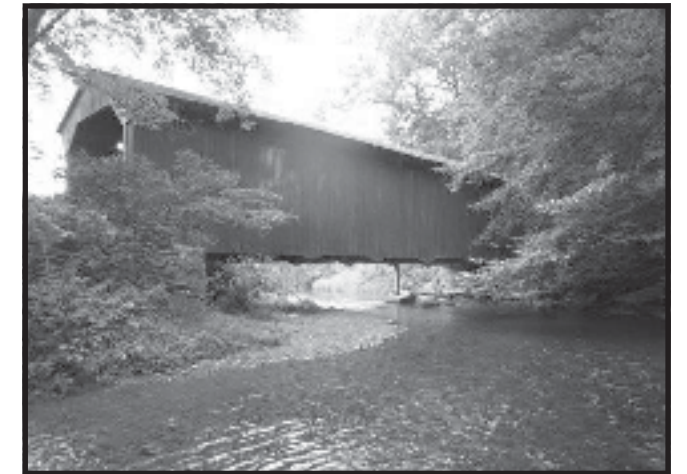
Mary Ann Pyle Bridge was built in 1881 and is listed on the National Historic Register
