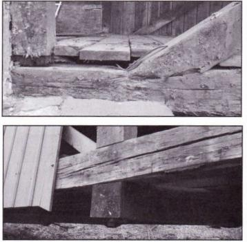
Photos by Frank Stroick show the damage to the supporting structure that will be repaired during the restoration project.
