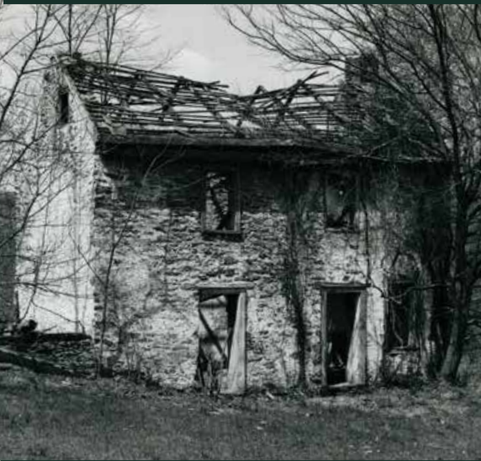
LAURELS FURNACE OFFICE
