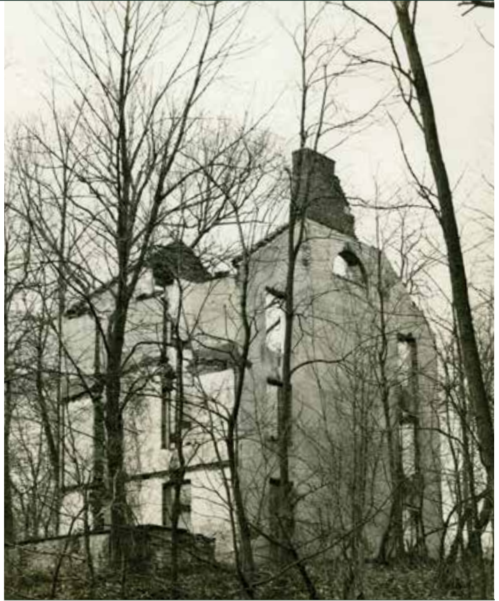
PLASTERED STONE HOUSE, LAUREL IRON WORKS
