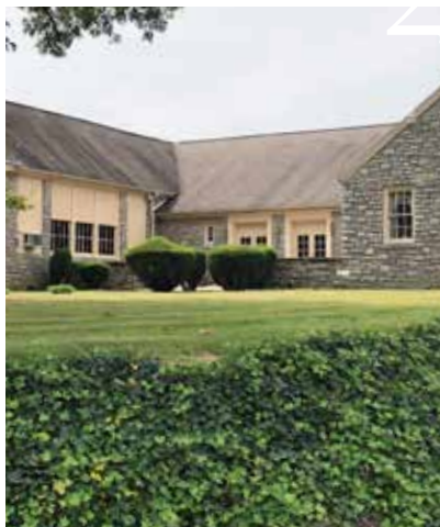
BRANDYWINE CONSERVANCY FIELD OFFICE HIGHLAND TOWNSHIP BUILDING
