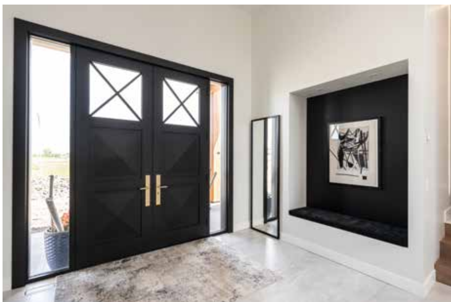
The 9' high wood doors, designed & crafted by Yarrow Sash & Door, lead to a foyer graced by equally dramatic large format ceramic tiles from Curtis Carpets. A convenient built-in bench is as elegant as it is functional.
