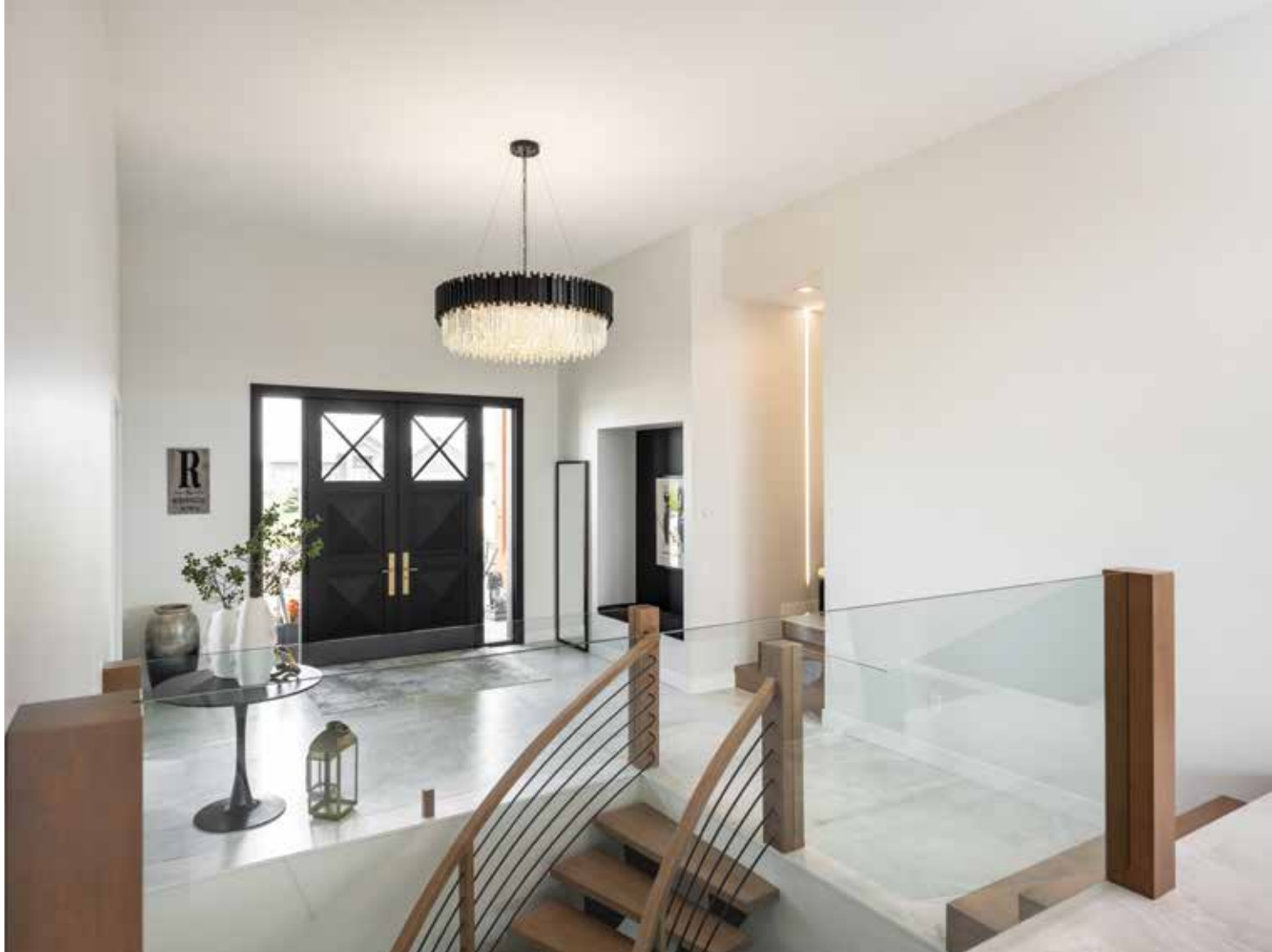
Leading down to the walkout basement, the curved staircase designed & built by Jake's Fancy Stair Work, features butcher-block treads, metal spindles & glass panels, for a clean modern look.
