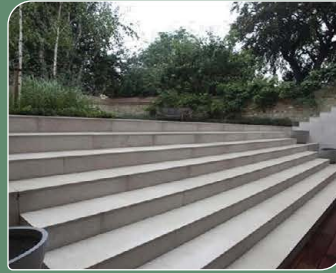
Concrete Entry Stairway at Honolulu Entry
