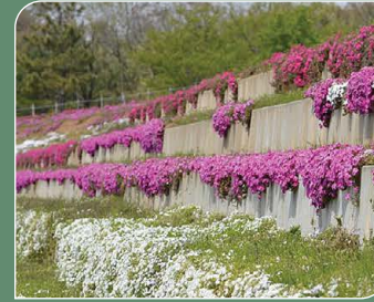
Garden Retaining Wall
