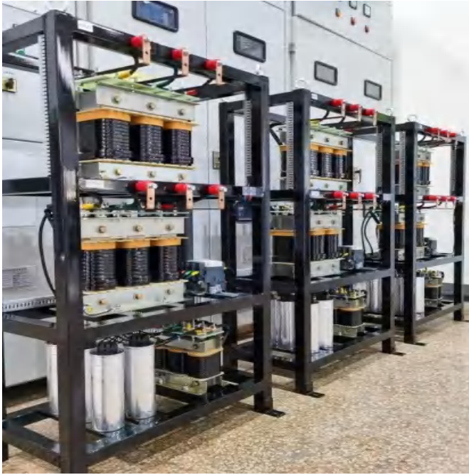
Passive Harmonic Filters
