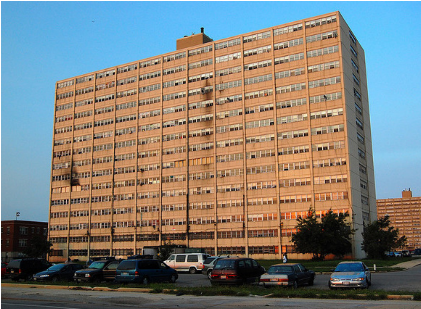
IMAGE 5. WITH A LIMITED BUDGET ON THEIR HANDS, CHA DESIGNED A HIGH-RISE SPREADING ACROSS THE AREA, WHICH ISOLATED THE INHABITANTS FROM THE SURROUNDING CONTEXT. THE PICTURE SHOWS ONE OF THE HIGH-RISES BEFORE DEMOLITION. ERIC ALLIX ROGERS, 2007.
