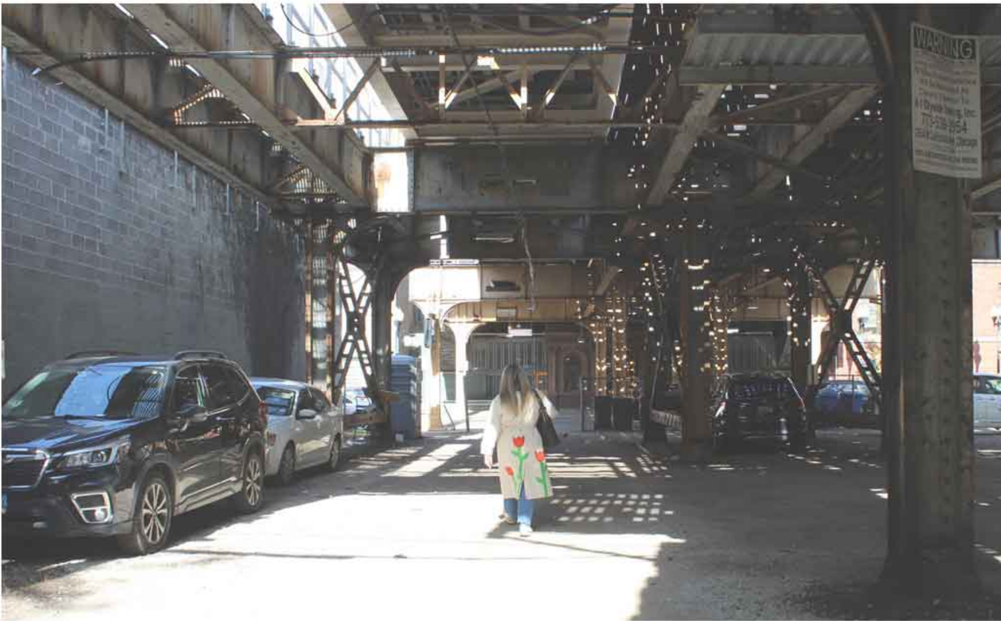
Looking West towards Sedgwick Station.
