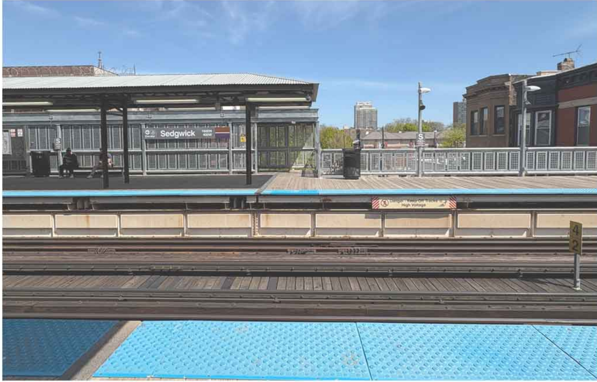
Loop-bound side of train platform.
