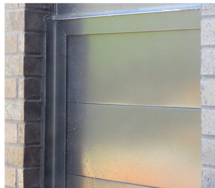
Image 47: Closeup of Cut Brick in Wall.
