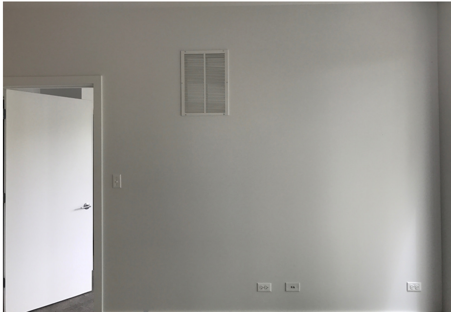
Image 30: 1620 Central Wall Closed Up.
