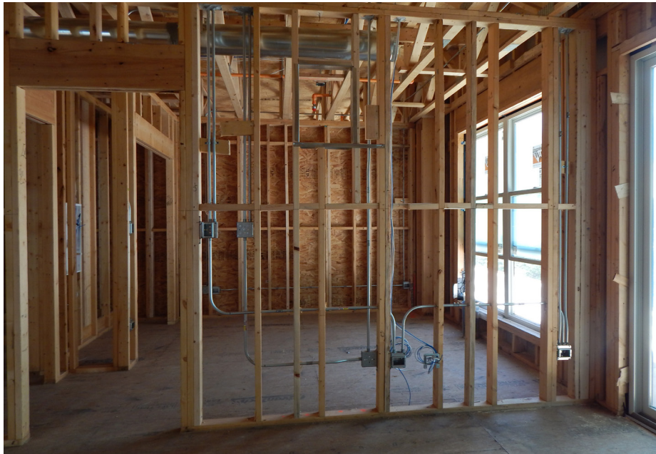
Image 28: 1620 Central Exposed Wall Framing.
