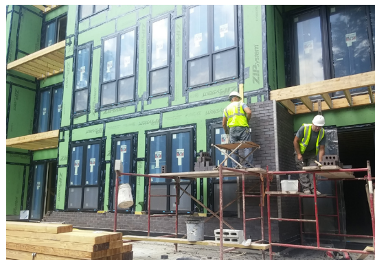
Image 36: Brick Installation at 1620. 4
