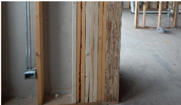
Image 12: Corner with 7 Additional Studs.
