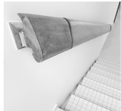
DETAIL | The break on the handrail acts as a tactile indication of the end of the treads. (International School in Annecy, France)
