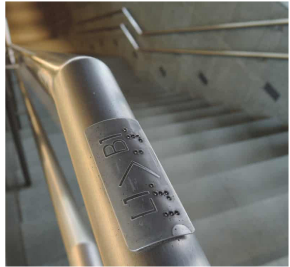
TACTILE HANDRAIL TAG | This tag presents both alphabet and braille of the floor level information via the sense of touch.
