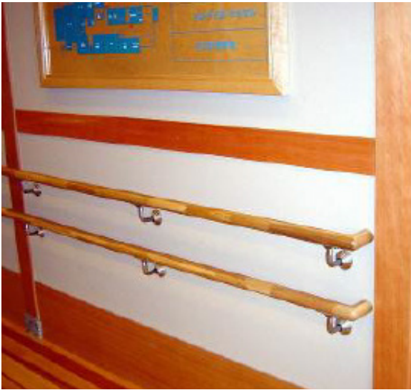
BI-LEVEL HANDRAIL | This design provide support for hand tracing technique that accomodates people with different hand levels with a material that is not cold to touch.
