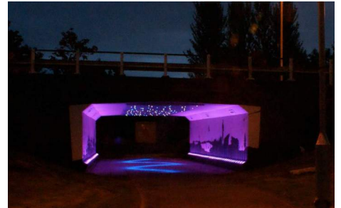
Craiglinn Underpass, Scotland 3
