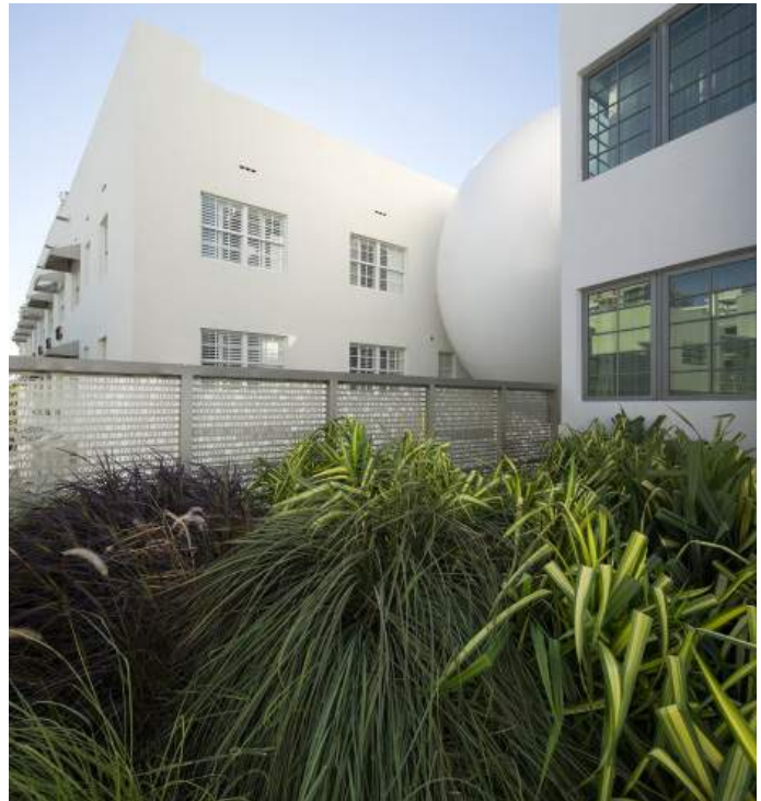
Fig. 14. The Betsy-Carlton Hotel, Shulman + Associates; Bridge design between historic building and new extension
