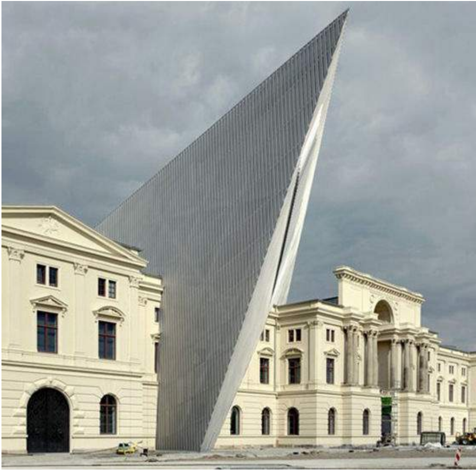
Fig. 13. Dresden's Military History Museum / Studio Libeskind. The new extension to the historic building cuts through the symmetry of building as a way to showcase the juxtaposition of tradition and innovation.
