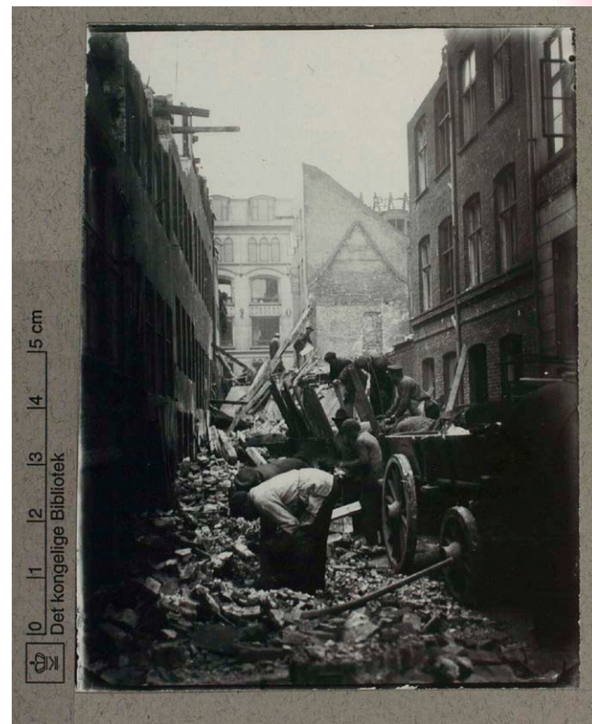
fig. 33 Demolition on Antonigade. Copenhagen, Denmark.
