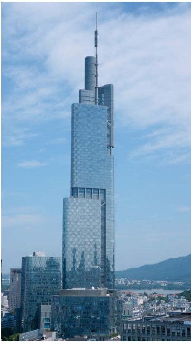
fig. 59 Zifeng Tower in Nanjing (450m). Nanjing, China. September 28, 2017.
