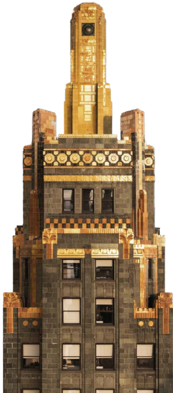
fig. 15 The Carbide and Carbon Building. Chicago, IL.
