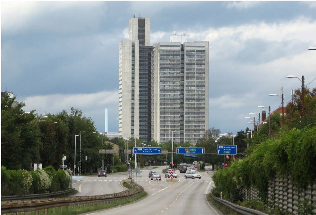
fig. 28 Herlev Hospital. Herlev, Denmark. August 2013.
