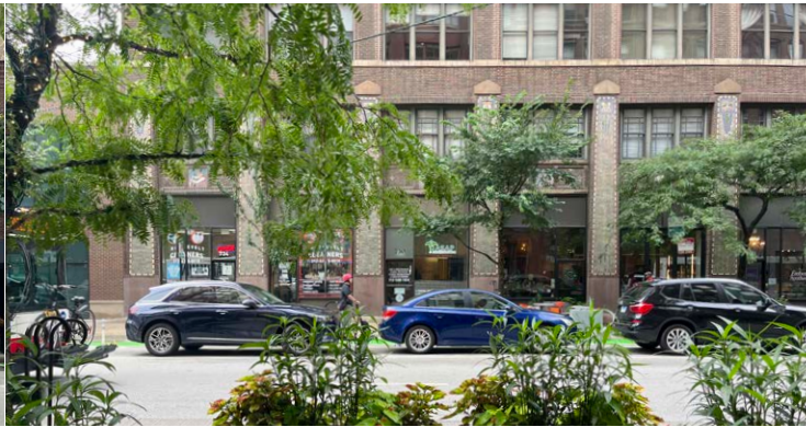
734 732 730 1912: George C. Nimmons, Franklin Building II (14 Floors)
