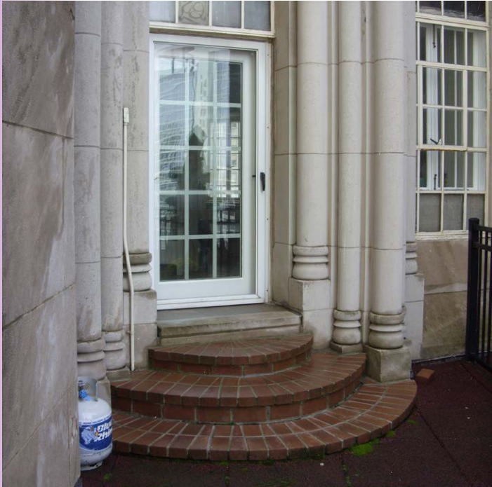
fig. 45 A red brick entryway to the penthouse of the pastor as part of the architecture meant to domesticate the tower. Chicago, IL. July, 2025.
