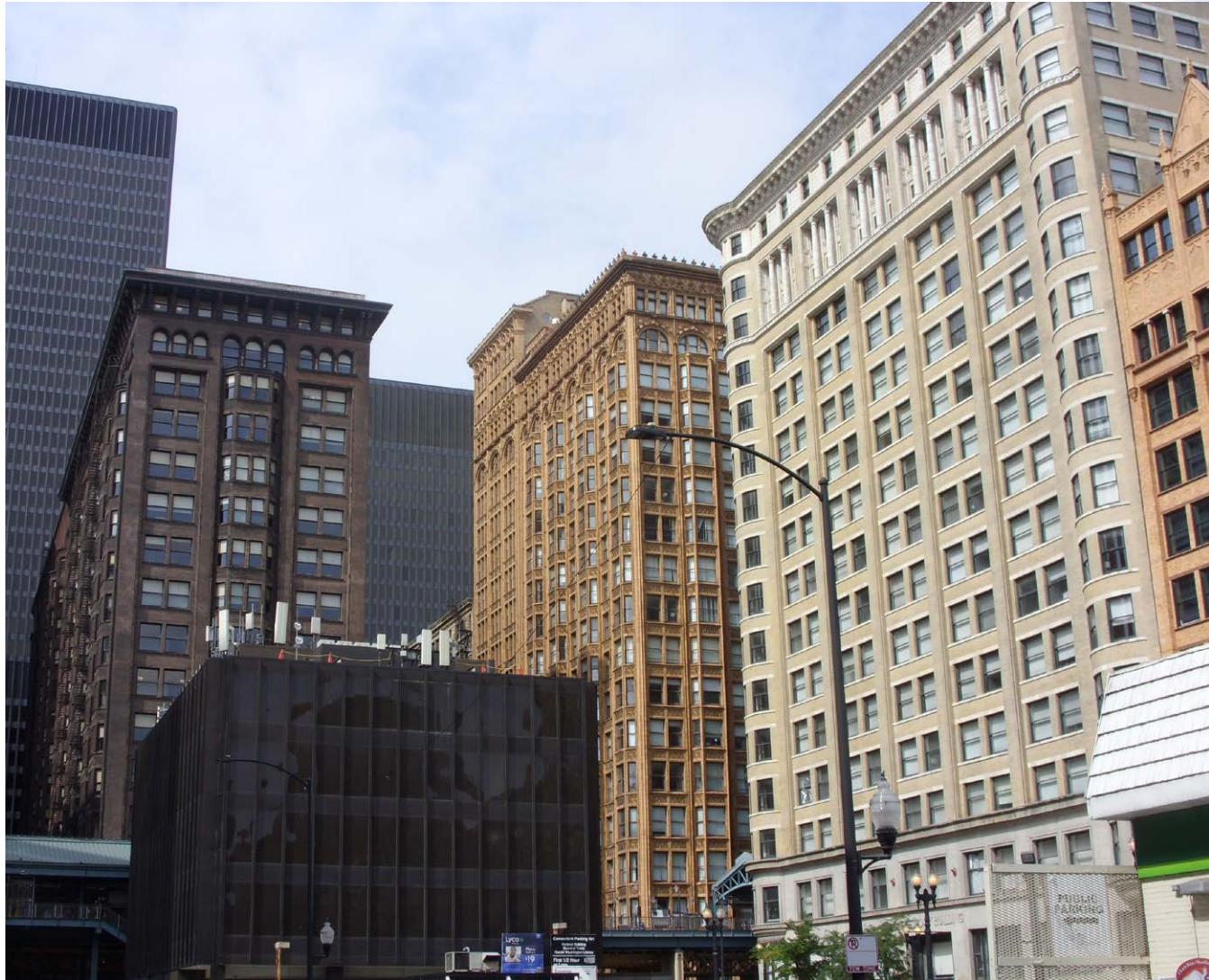
fig. 10. Monadnock & Fisher Building. Chicago, IL. July 2025.
