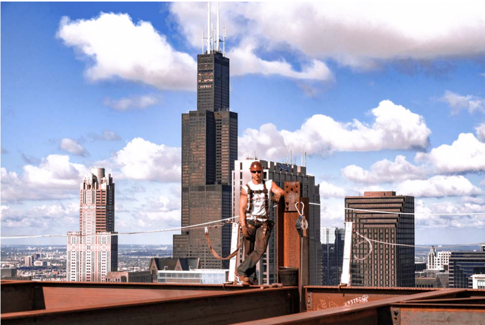
fig. 5 Steel worker in Chicago. Chicago, IL. August 2008.
