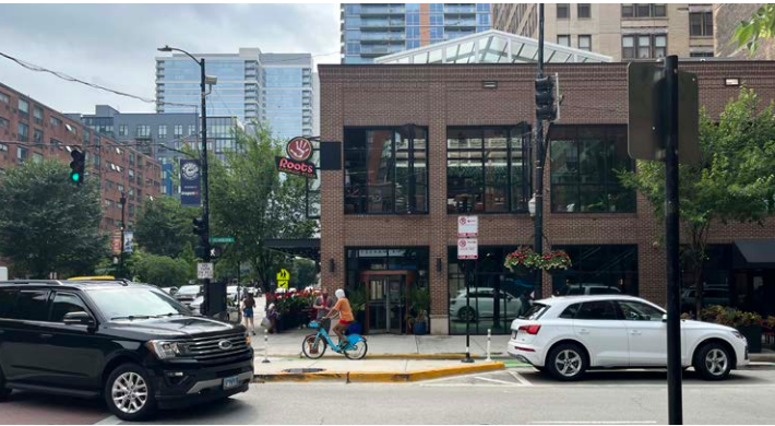
S Dearborn St. & Polk St. 744 2020: Myefski Architects (2 Floors) 742
