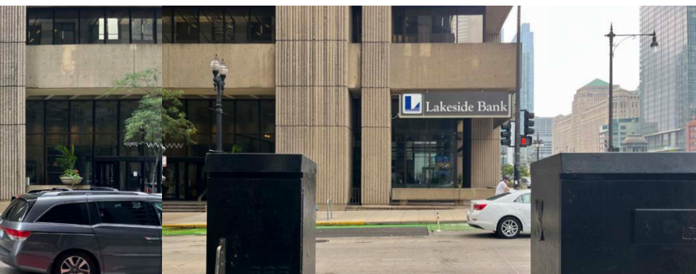
1968: C.F. Murphy Associates, Blue Cross-Blue Shield Building (78m, 16 Floors)
