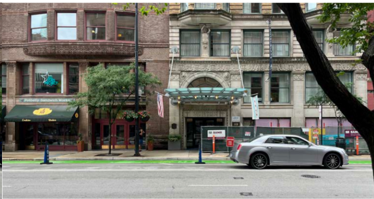
538 1896: William Le Baron Jenney & Charles Mundie, Morton Building (12 Floors)
