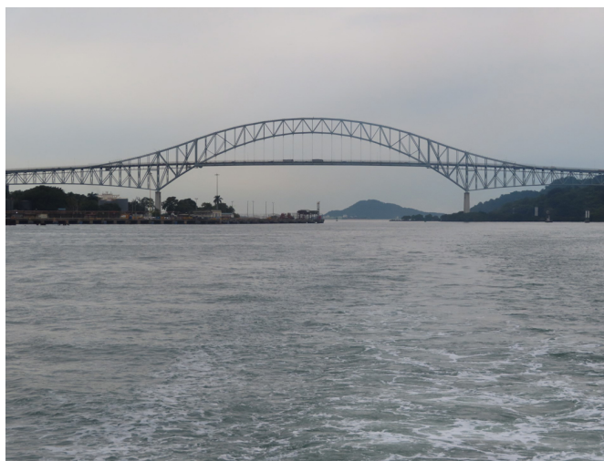
Figure 27. The Pan-American bridge over the Panama Canal. Photo Credit: Pam Olson.
