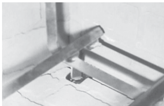
Figure 7.3 Grate Secured In Grate Bracket
