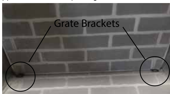
Figure 7.2 Grate Brackets In Place
