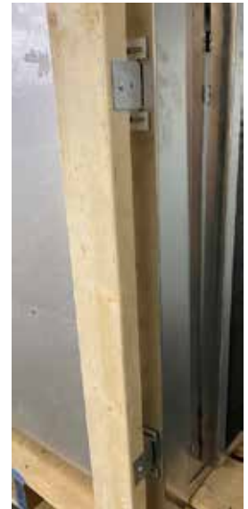
Figure 6.8 Fasten installation brackets to wall framing
