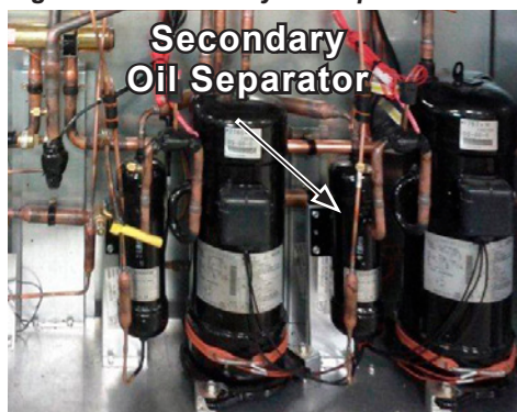
Figure 18: Secondary Oil Separator
