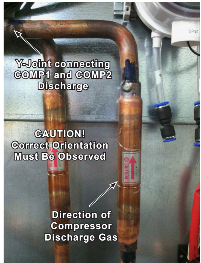
Figure 19: Discharge Line Check Valves on Large Cabinet (7.5T) Heat Pump (DPH)
