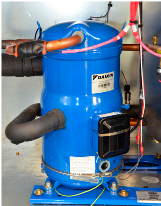
Figure 27: Compressor Suction and Discharge on DPS 025–028 units
