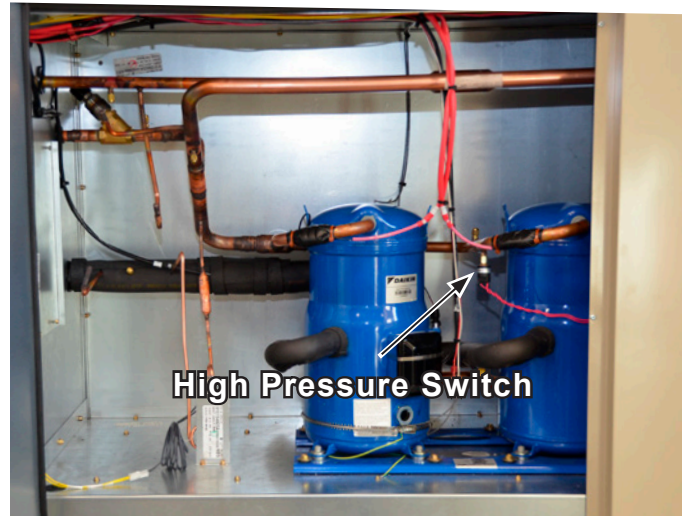
Figure 28: High Pressure Switch
