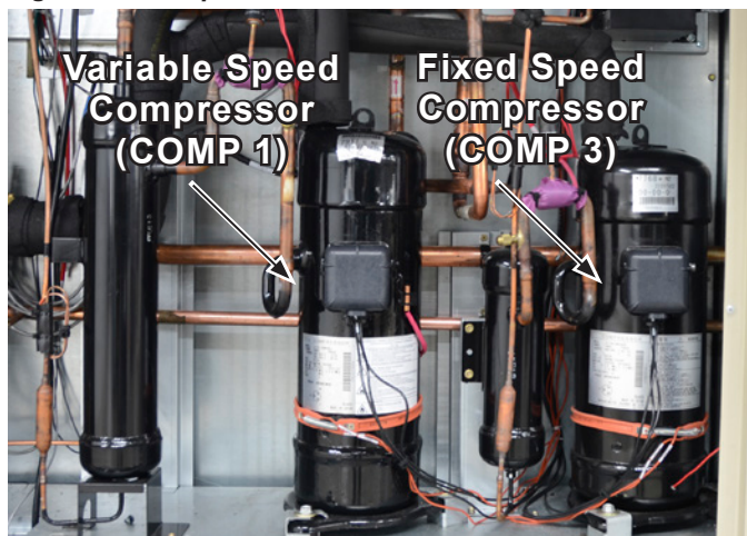
Figure 15: Compressor Tandem on Medium Cabinet
