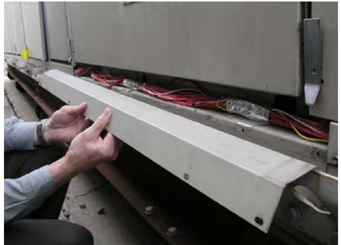
Figure 52: Control Wiring Raceway
