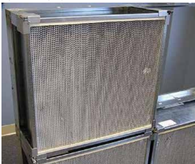
Figure 26: Properly Installed Filter Inside of the Frame
