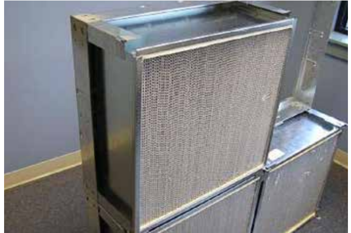
Figure 22: Filter Placed Inside of Frame
