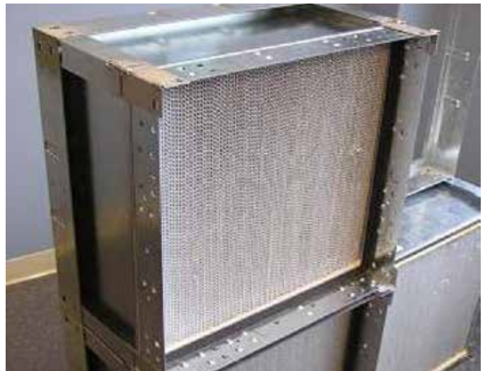
Figure 31: Properly Installed HEPA Filter
