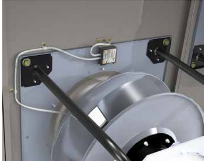
Figure 75: Piezometer Transducer
