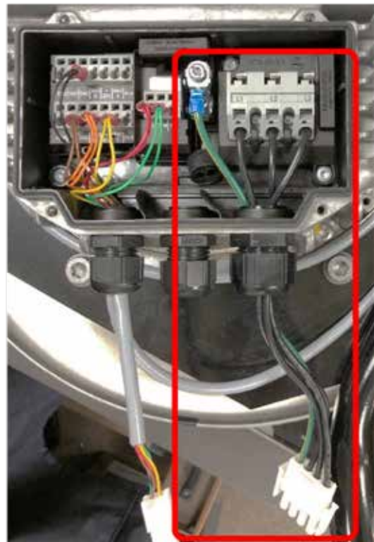
Figure 67: Fan - High Voltage Wiring
