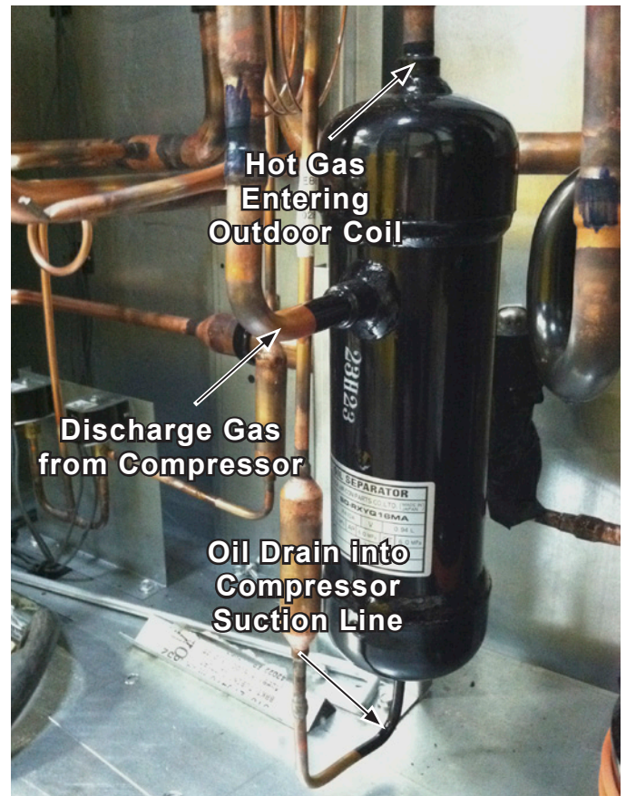
Figure 22: Oil Separator
