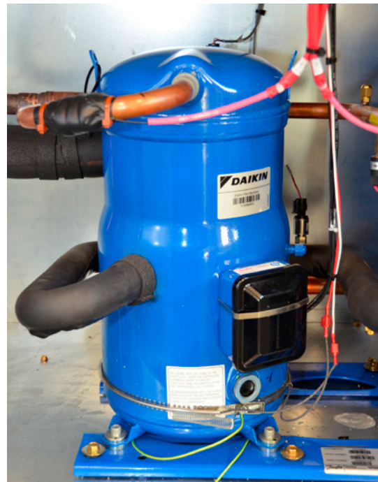
Figure 32: Compressor Suction and Discharge on DPS 025–028 units
