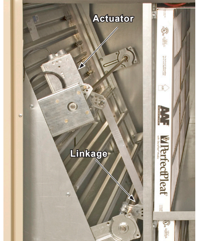
Figure 11: Damper Assembly
