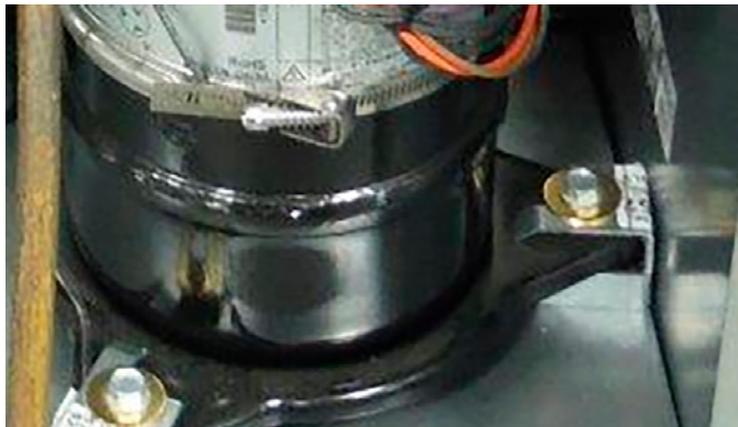
Figure 18: Compressor Brackets
