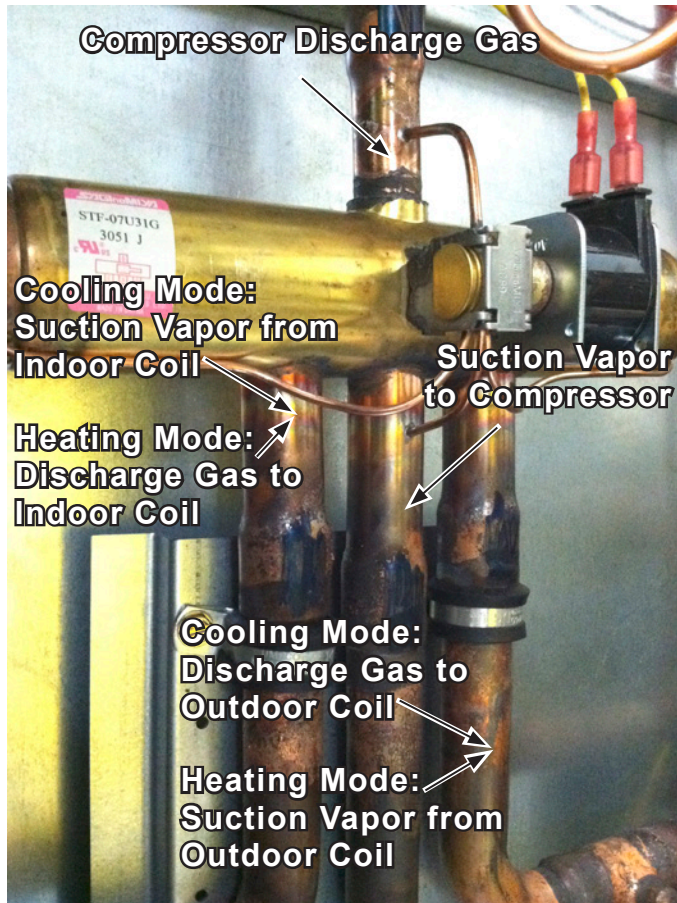
Figure 27: Four-Way Valve
