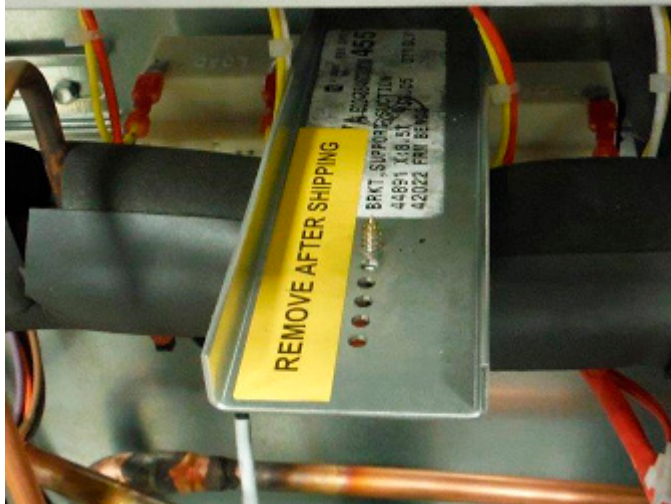
Figure 18: Compressor Brackets
