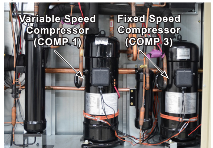
Figure 20: Compressor Tandem on Medium Cabinet
