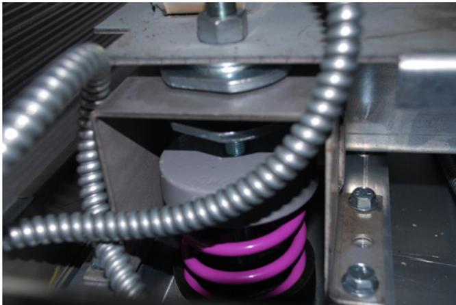
Figure 75: RDT Spring Mount Hold-Down Fasteners
